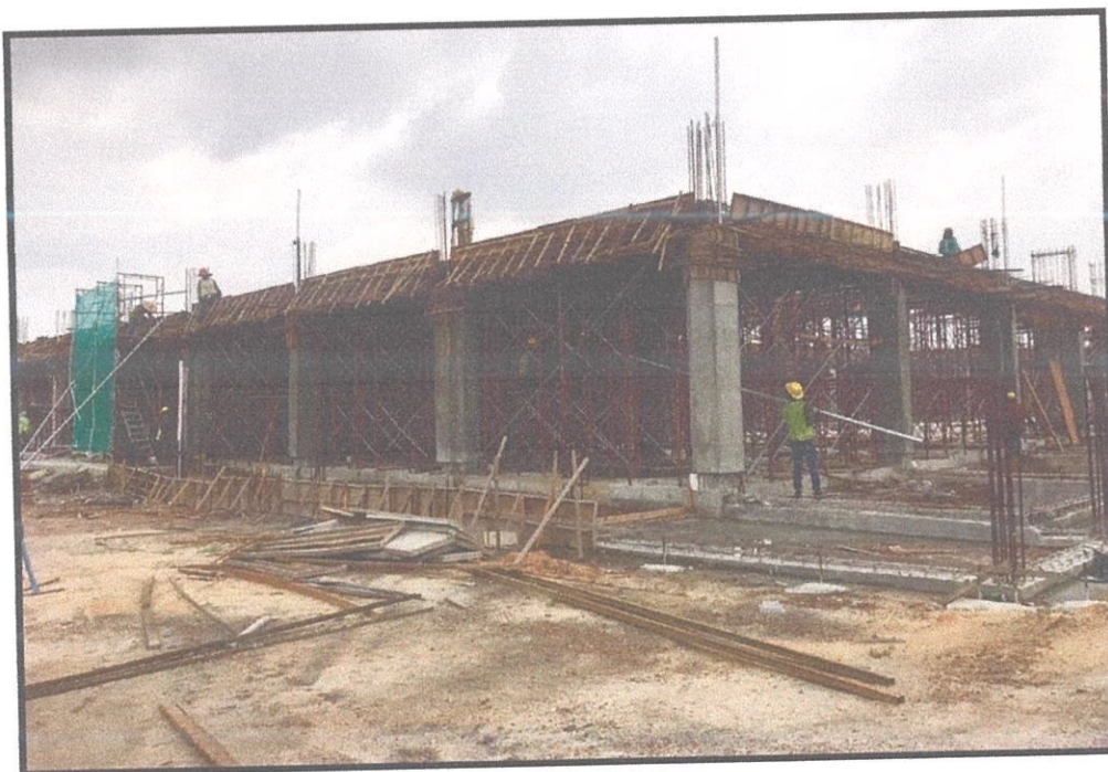
Photo 3.1: Project Progress to date 29/10/2018
