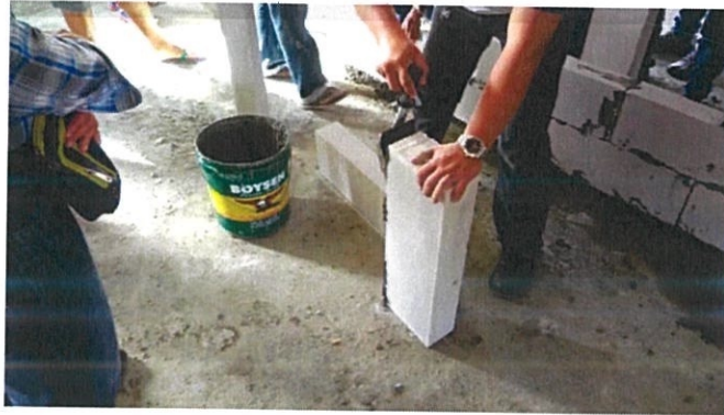
PHOTO 3.22 : Apply adhesive on block
