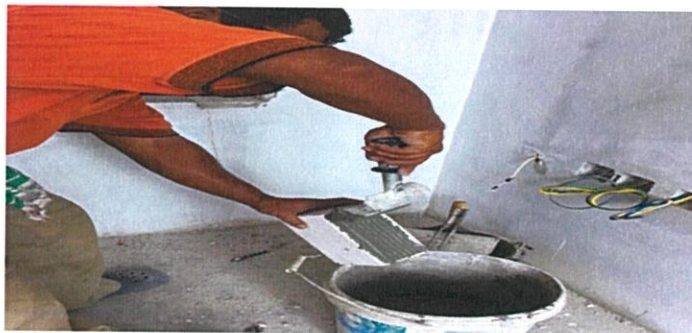
PHOTO 3.17 : Laying adhesive
