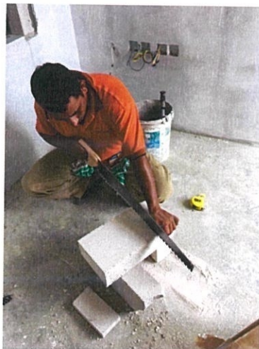
PHOTO 3.21 : Cut the block with saw
