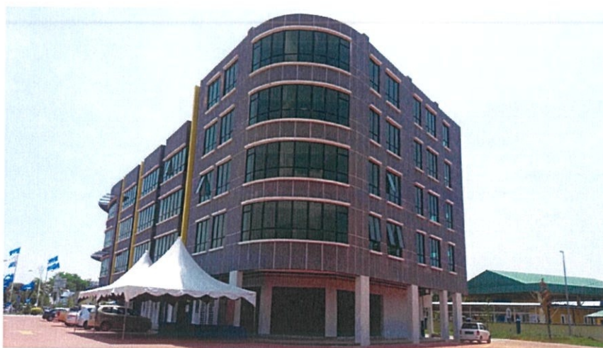
Photo 3.1 : Front View of Hotel Bajet
