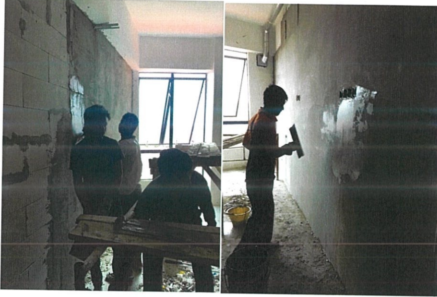
PHOTO 3.26 : Plastering work
