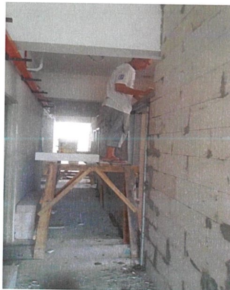
PHOTO 3.25 : Install block at the slab
