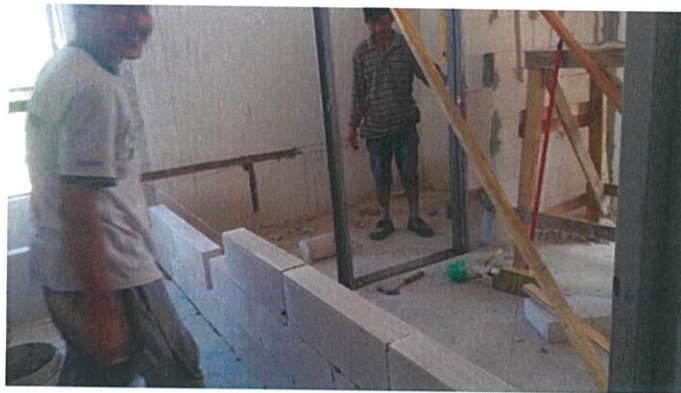
PHOTO 3.23 : Alignment string move upward
