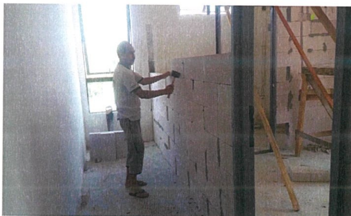
PHOTO 3.18 : Tap with rubber mallet
