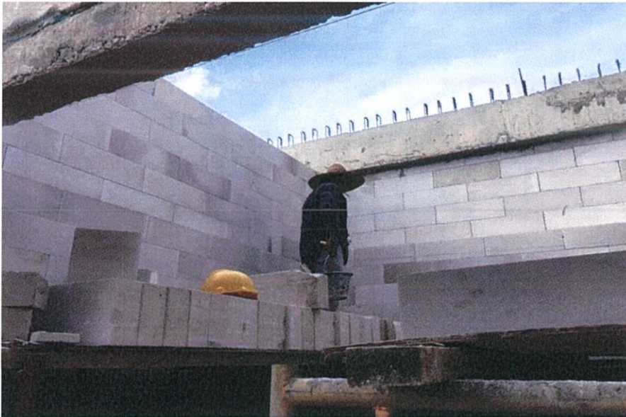
Figure 3.6 Workers installing AAC blocks
