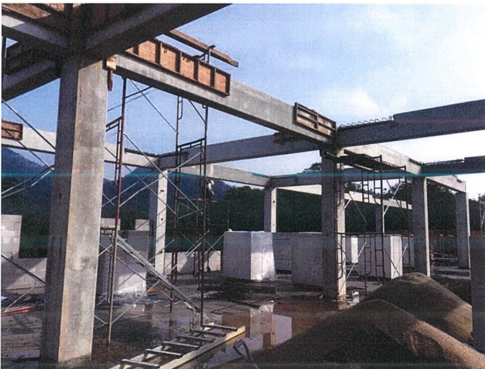
Figure 3.4 Framed structure of Industrialised Building System (IBS)
