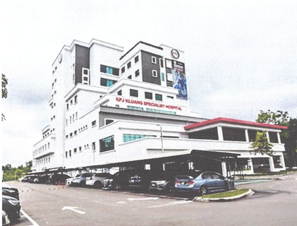
Figure 3.3: The New Buildings Of KPJ Kluang Specialist Hospital
