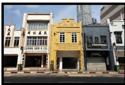
Figure 4: Art Deco Shophouses (Source: Shang, 2019)
