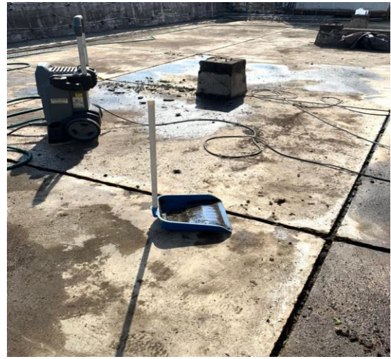
Helped to clean the rooftop
