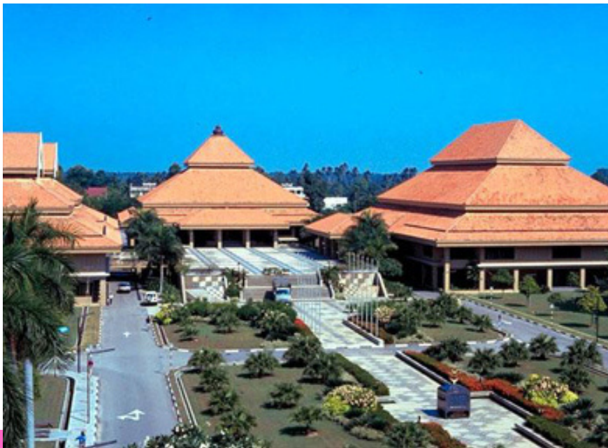
Photo 3.4 Rectangular wooden buildings "Opis Pohon Celagi"
