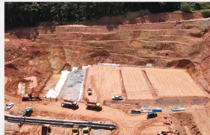
Slope Protection Work
