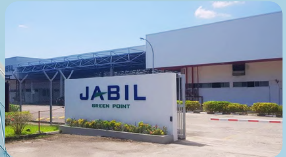
Plant Bukit Minyak Warehouse
