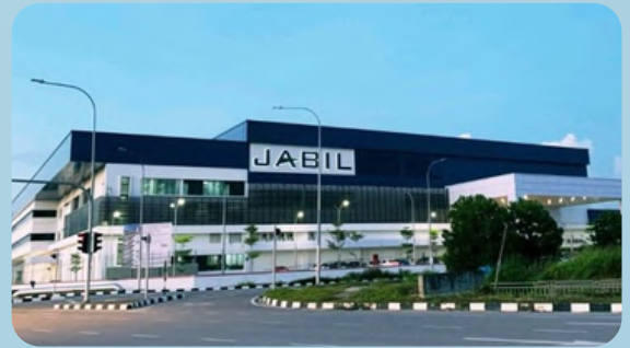
Plant Batu Kawan
