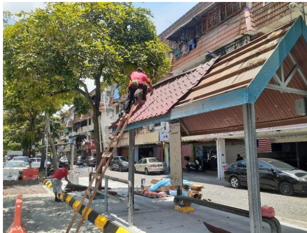
Figure 13 shows the demolishing of roof structure.
