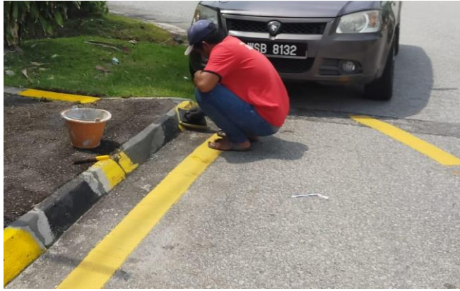
Figure 12 shows the worker is painting the kerbs.
