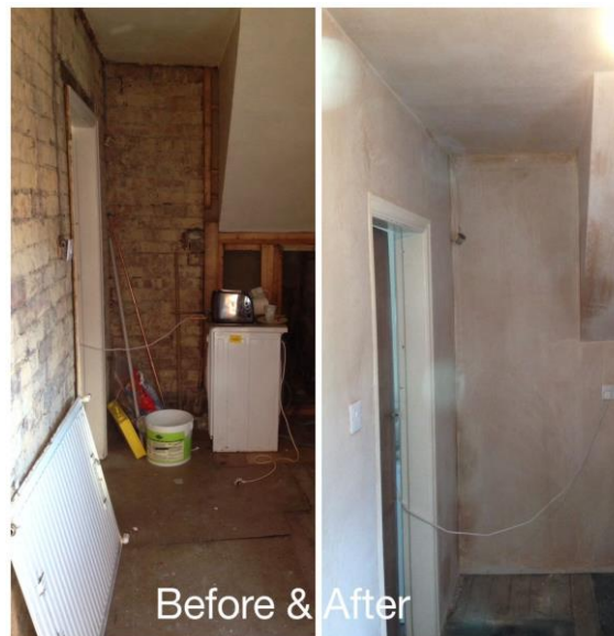
Figure 3.2.2 above shows before and after plastering.
