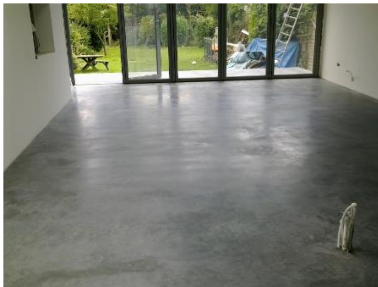
Figure 3.3.2 above shows the concrete floor.
