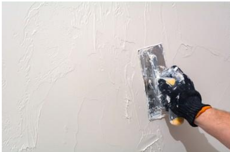
Figure 3.2.1 above shows plastering the wall
