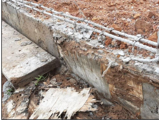
Figure 3.19: Expanded Ground Beam's Concrete.
