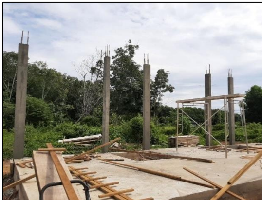
Figure 3.16: The Column That Has Been Dismantle.
