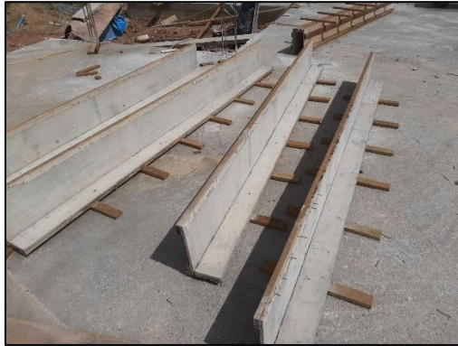
Figure 3.13: The Column's Formwork That Has Been Form.
