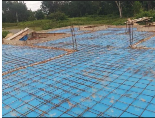
Figure 3.8: Installed BRC on DPM Layer.
