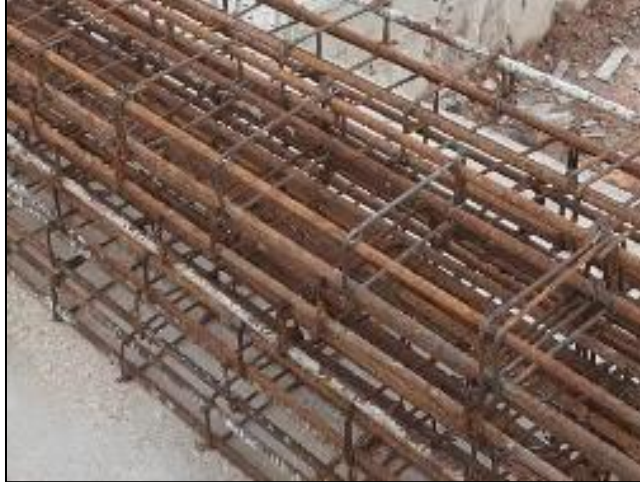
Figure 3.23: R6 Steel Reinforcing Link Bonded Together with Y12 Steel Bar.
