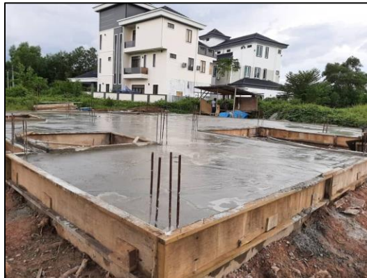
Figure 3.9: Freshly Poured Concrete.
