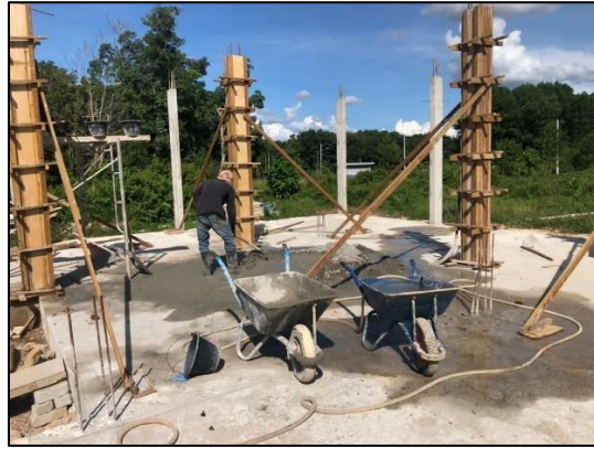
Figure 3.15: The Concrete Was Mixed by the Worker.
