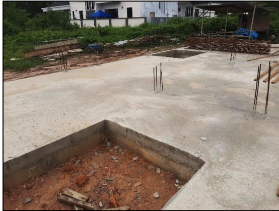
Figure 3.10: Concrete Slab That Has Been Cure.
