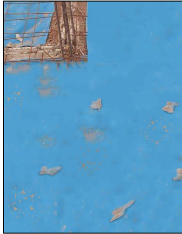
Figure 3.6: DPM Layered on The Compacted Soil.
