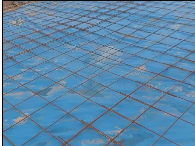
Figure 3.24: Installed BRC on DPM Layer.
