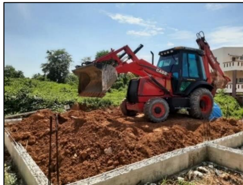
Figure 3.5: Backhoe Was Backfilling the Soil.
