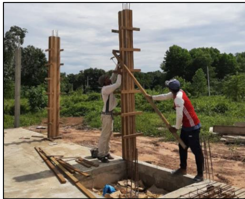
Figure 3.14: The Column's Formwork Were Installed by the Workers.
