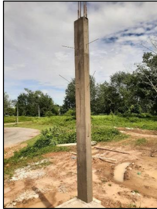
Figure 3.17: Concrete Column That Has Been Cure.
