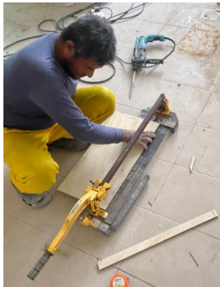
Figure 10 Using Cutting Tiles Machine
