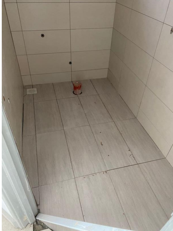
Figure 13 Finished Product of Installed Tiles for Master Bathroom
