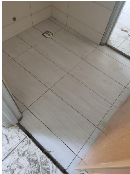
Figure 11 Finished Product of Installed Tiles for Bathroom 2
