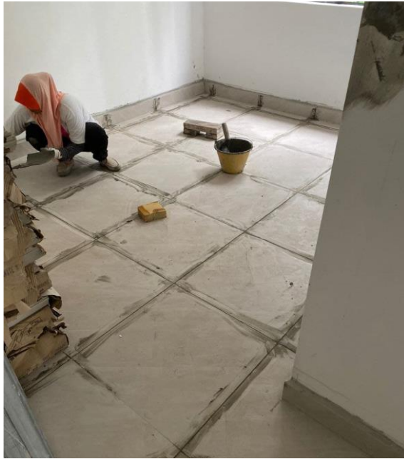
Figure 15 Grouting for Bedroom 2 Ceramic Tiles
