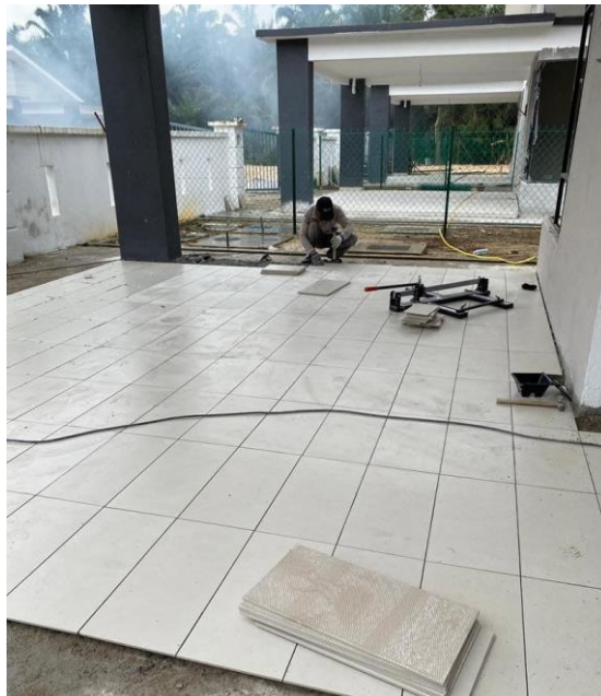
Figure 21 Installation of Tiles for Car Porch
