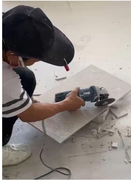
Figure 9 Using Angle Grind Machine
