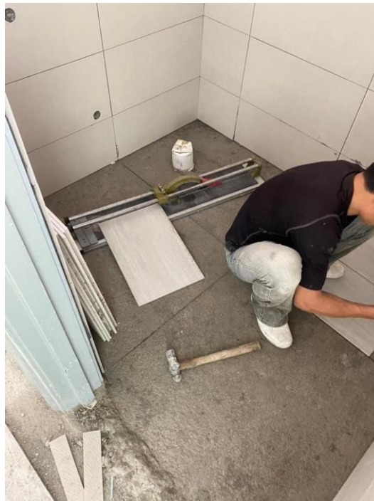
Figure 12 Installation of Ceramic Tiles in Kitchen Bathroom
