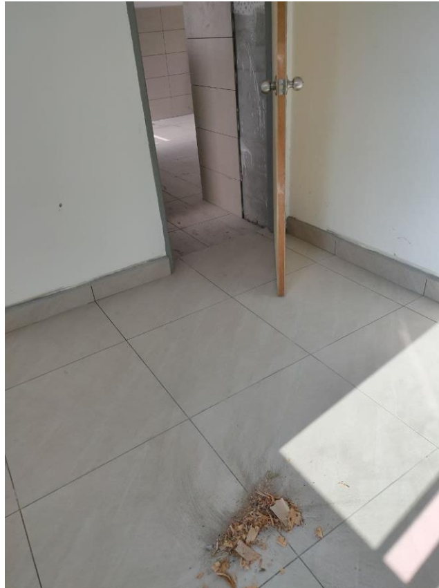
Figure 17 Finished Product of Installed Tiles for Storage Room
