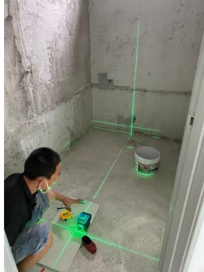
Figure 7 Marking Alignment for Tiles
