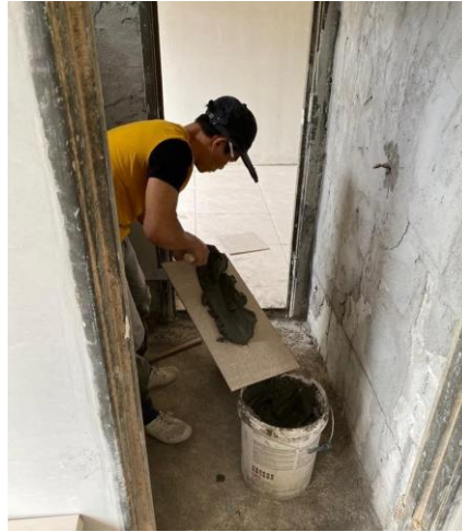
Figure 8 Spreading Adhesive on a Tile
