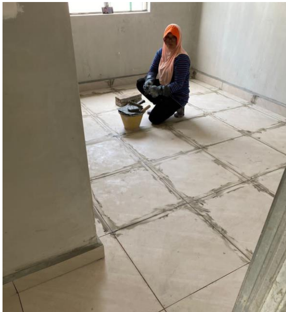
Figure 16 Grouting for Bedroom 3 Ceramic Tiles
