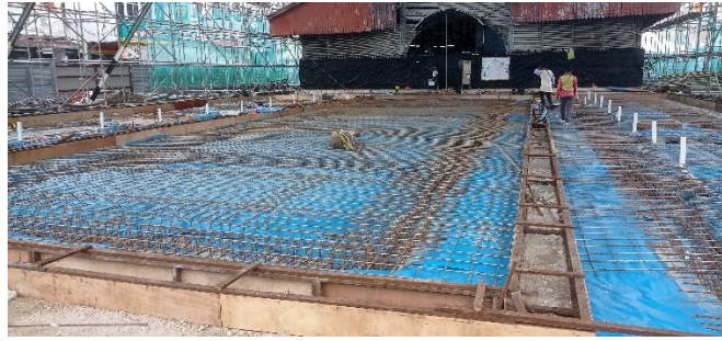
Figure 3.2.5 (Laying brc mesh)
