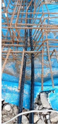
Figure 3.2.6 (HDPE pipe were used for the internal cold water plumbing system)
