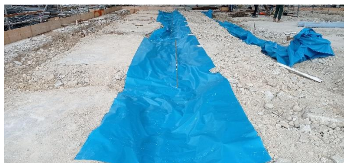
Figure 3.2.5 (Applying dpm in the excavated area)
