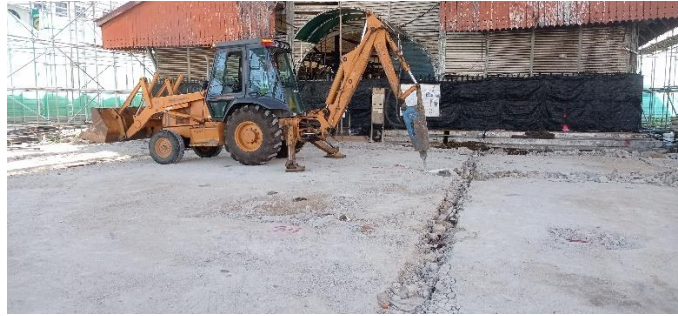
Figure 3.2.4 (Backhoe breaker is used to break the ballast)
