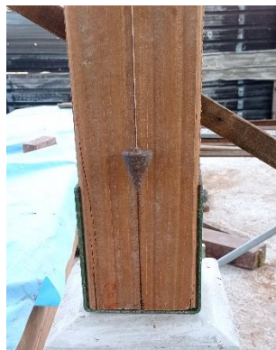
Figure 3.2.7 (Using a plummet to check the wood straightness)
