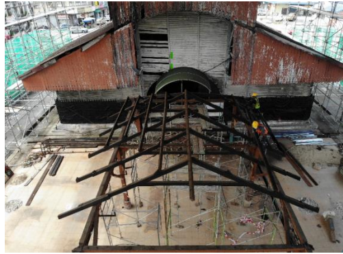
Figure 3.2.1 (arked siang malam being disassembled)
