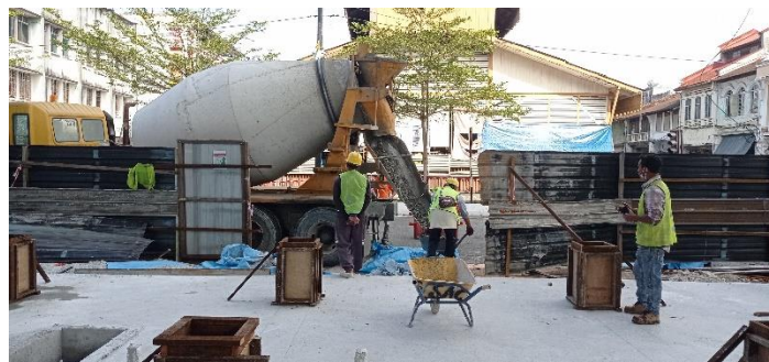
Figure 3.2.7 (Pouring concrete)
