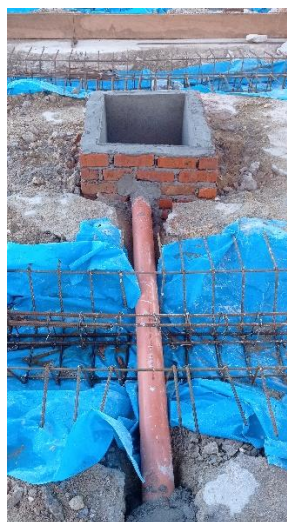
Figure 3.2.6 (Pipe UPVC were used for water outlet to the perimeter drain)
