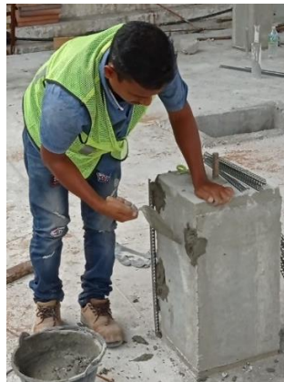
Figure 3.2.7 (Putting corner bead)
