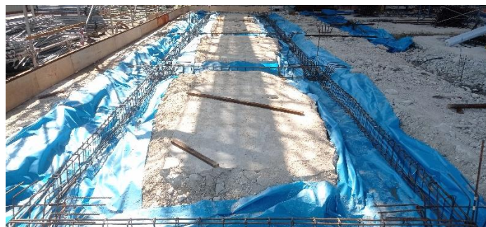
Figure 3.2.5 (Installing steel bar for beam slab in the raft footing)
