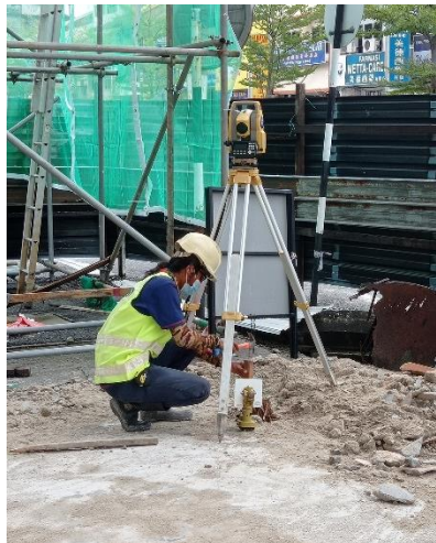
Figure 3.2.3 (Column pegging)
