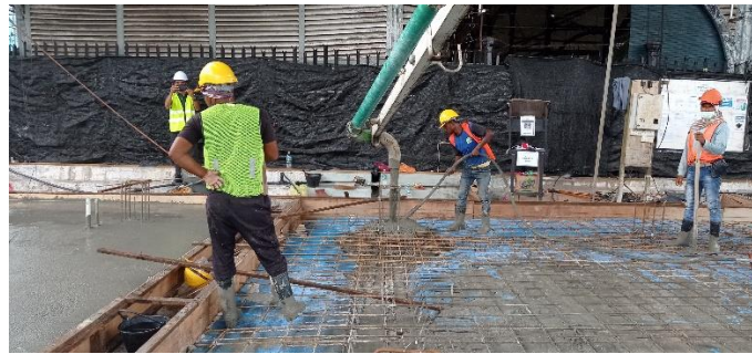
Figure 3.2.5 (Pouring concrete)
