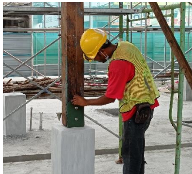
Figure 3.2.7 (Checking the wood column uphold)
