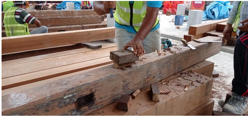
Figure 3.2.7 (Patching wood)
