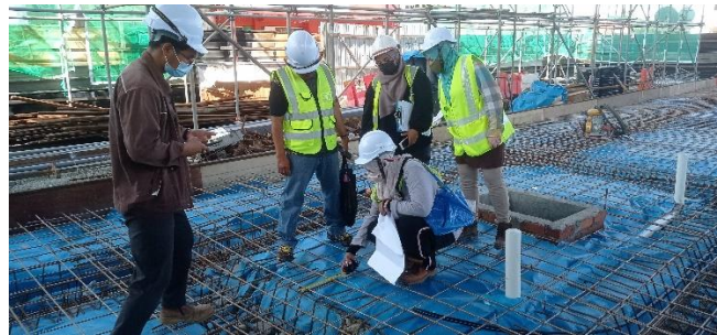
Figure 3.2.5 (Taking lapping measurement of brc mesh)
