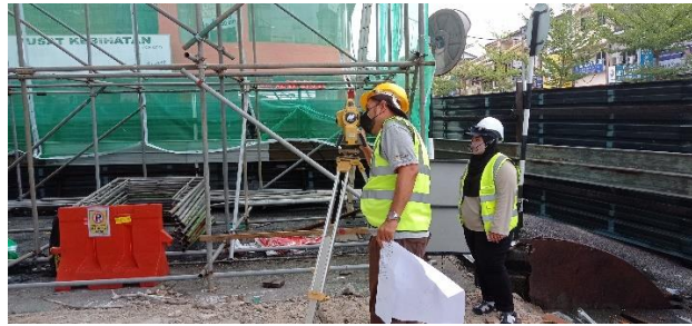
Figure 3.2.3 (Pegging work in progress)
