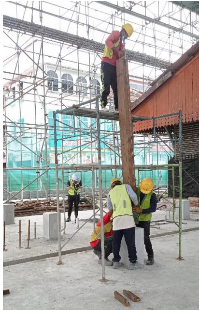
Figure 3.2.7 (Installing wood column)
