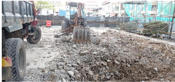
Figure 3.2.4 (Digging up debris using back hoe)
