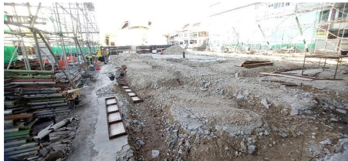
Figure 3.2.4 (Ballast completely excavated according to the building grid line)
