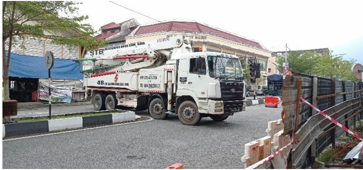
Figure 3.2.5 (Pump truck used to pour concrete into the construction site)
