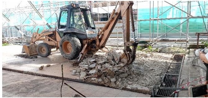
Figure 3.2.2 (Backhoe is used to excavate tiles)
