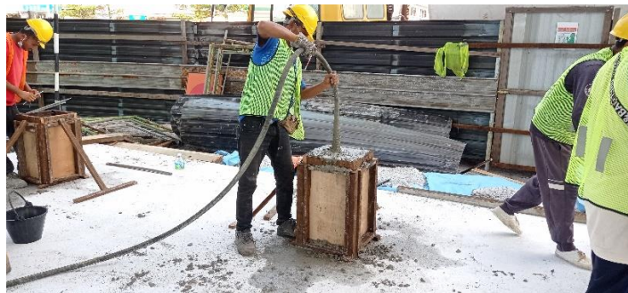
Figure 3.2.7 (Using vibrator to shake the concrete)
