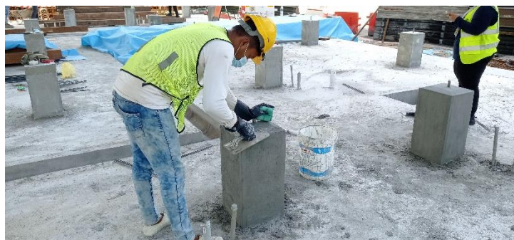
Figure 3.2.7 (Plastering concrete stump)
