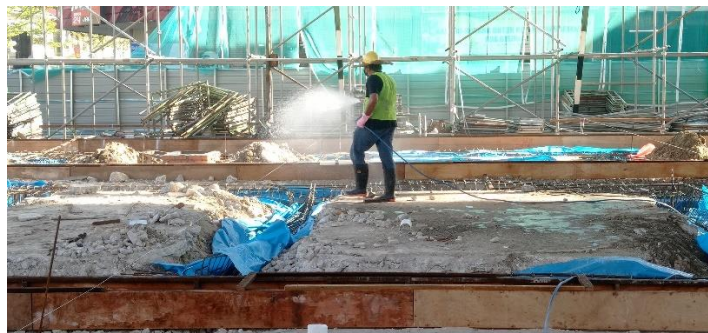
Figure 3.2.5 (Spraying anti-termite)
