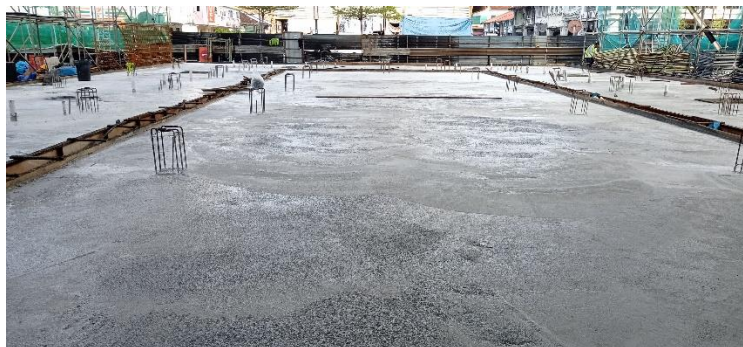
Figure 3.2.5 (Hardened concrete slab)
