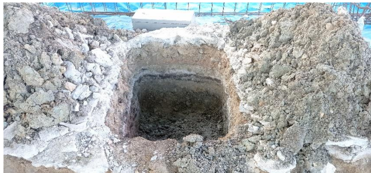
Figure 3.2.6 (Hacking and digging the ground for grease trap hole)
