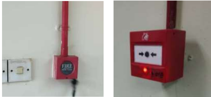
Figure 3.5: Manual call point/break glass.
