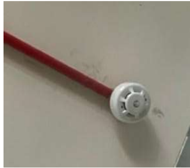
Figure 3.3: Heat detector
