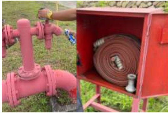
Figure 3.27: fire hydrant
