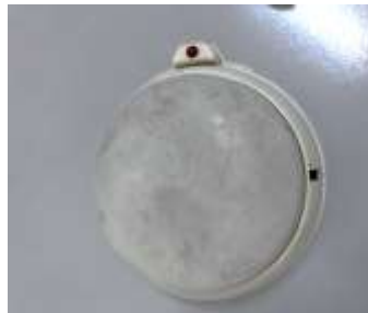
Figure 3.4: Smoke detector.
