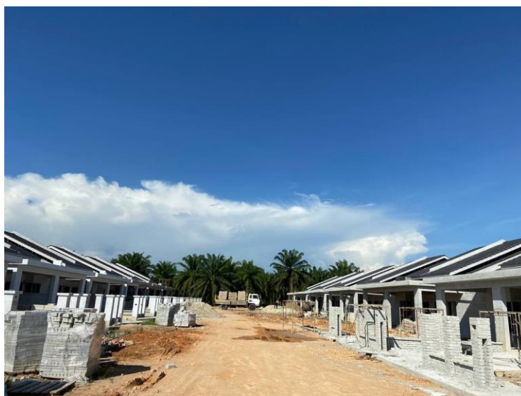
Figure 3.2: Linggi Idaman site
