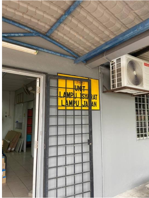
Figure 1.1: JKR streetlight department
