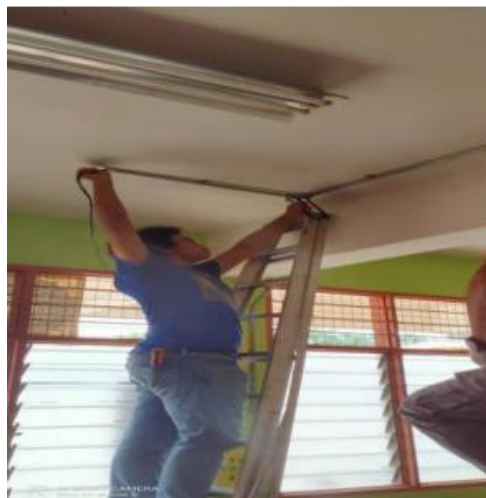
Figure 3.1 (1): Rewiring works for lamp in classroom
