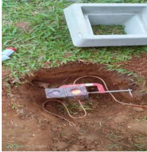
Figure 3.1 (4): Underground cable installation work
