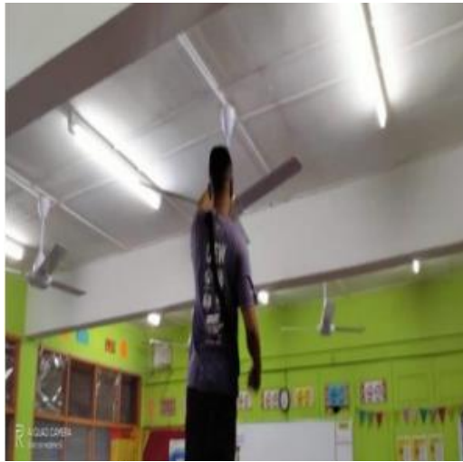
Figure 3.1 (2): Rewiring works for fans in classroom
