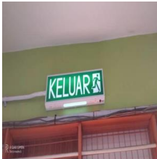
Figure 3.1 (3): Rewiring works for EXIT LED sign
