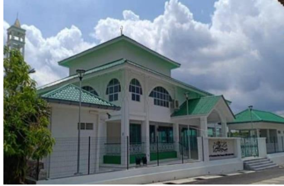
Figure 6: Mosque, Tampoi, Johor Bahru, Johor.
