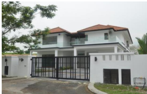
Figure 17: Front elevation bungalow, Jalan Perindu 1, Ledang Heights.
