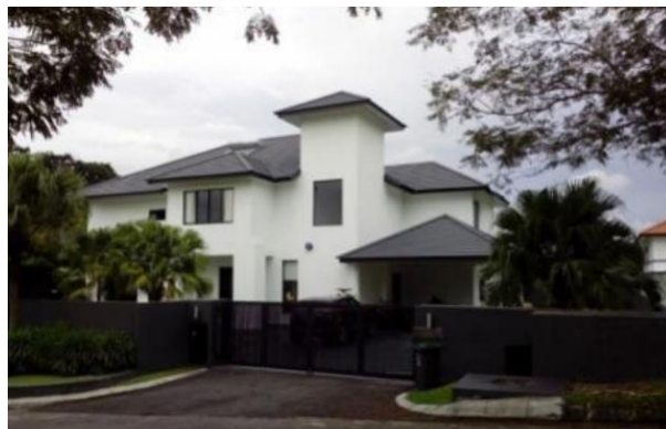
Figure 14: Front elevation bungalow, Jalan Perindu 3, Ledang Heights.
