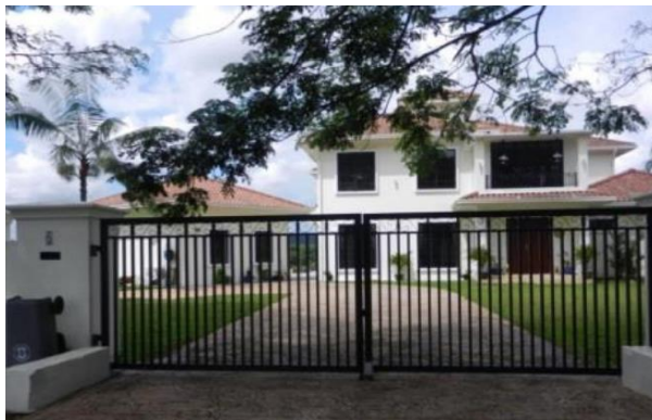
Figure 11: Front elevation bungalow, Leisure Farm, Pulau.
