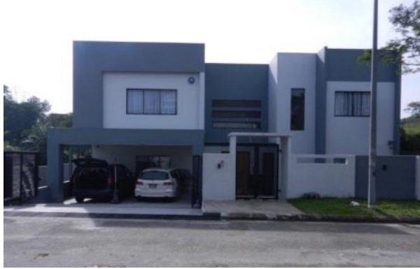
Figure 9: Two storey bungalow, Jalan Perindu 1, Ledang Heights.
