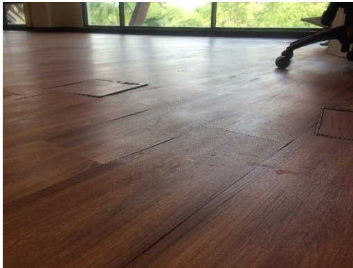
Figure 3.4.9 The peaked vinyl planks
