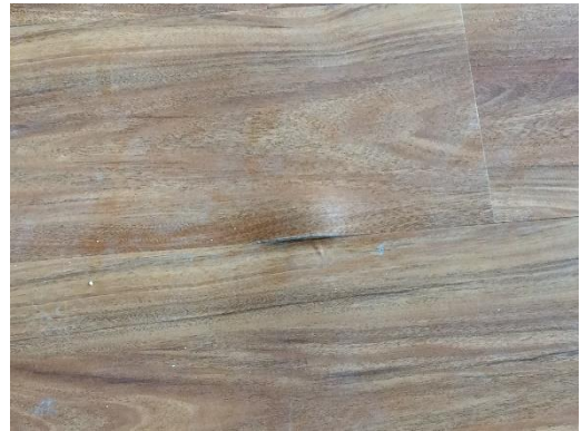
Figure 3.4.10 The warped vinyl plank
