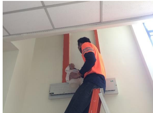
Figure 3.4.8 Wiping the paint stains using thinner
