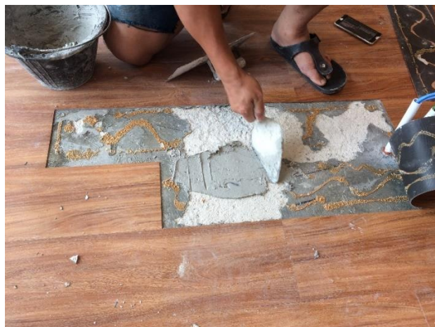
Figure 3.4.11 Skim work on uneven cement floors
