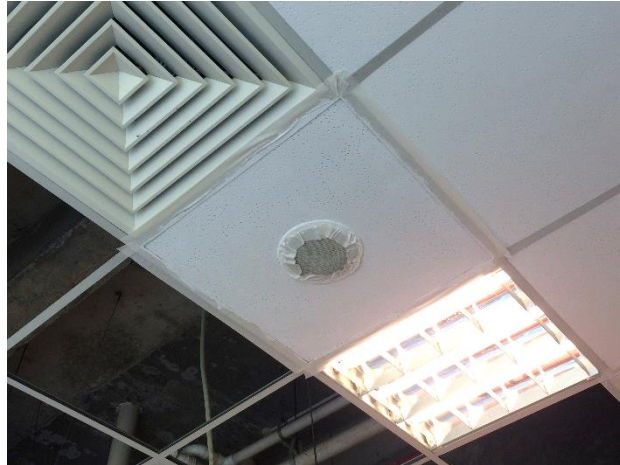
Figure 3.4.6 The appearance of the ceiling after painting with masking tape on
