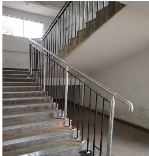
Figure 3. 18: The example of railing staircase
