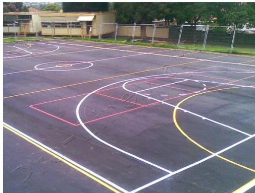
Figure 3. 26The example for area court marking
