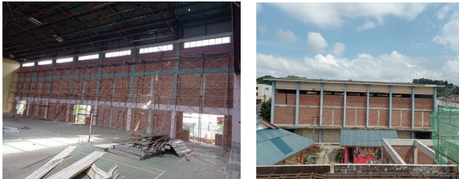
Figure 3. 11: The view in a construction site after masonry work
