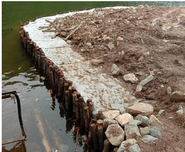
*Figure 3.2.11 An ideal arrangement of mangrove piles*
