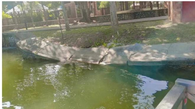
*Figure 1.3 The site collapsed because the soil had settled into the water*
