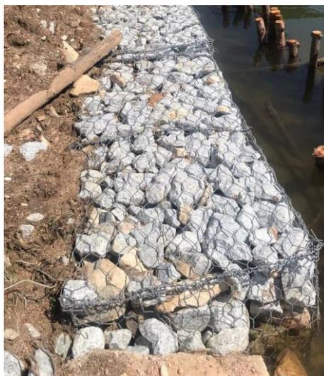
*Figure 3.2.8 Gabion cage and rock inside it*
