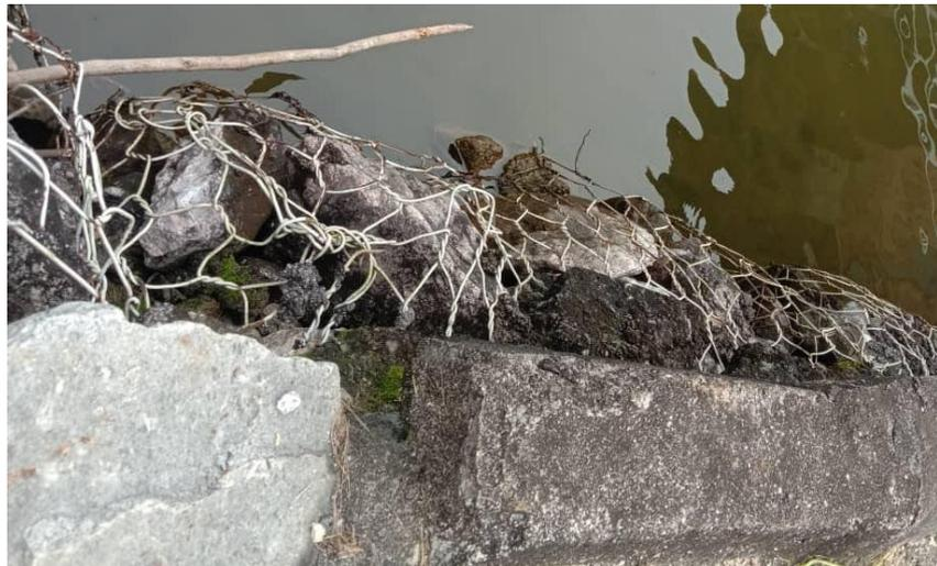
*Figure 3.2.3 Gabion that broken*
