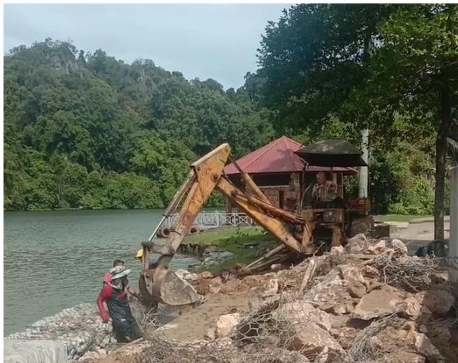
*Figure 3.2.7 Backhoe's operator put the new rocks near the edge island*
