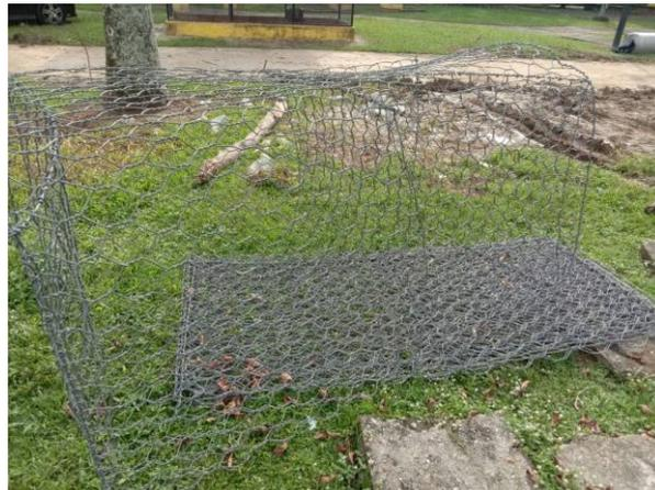
*Figure 3.3.2 Gabion cage*
