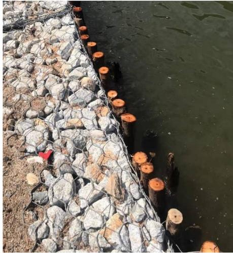
*Figure 3.2.10 The way mangrove piles should be arranging*
