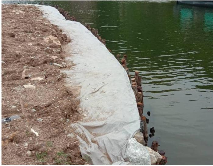
*Figure 3.2.9 Non-Woven Geotextile as cover of gabion*
