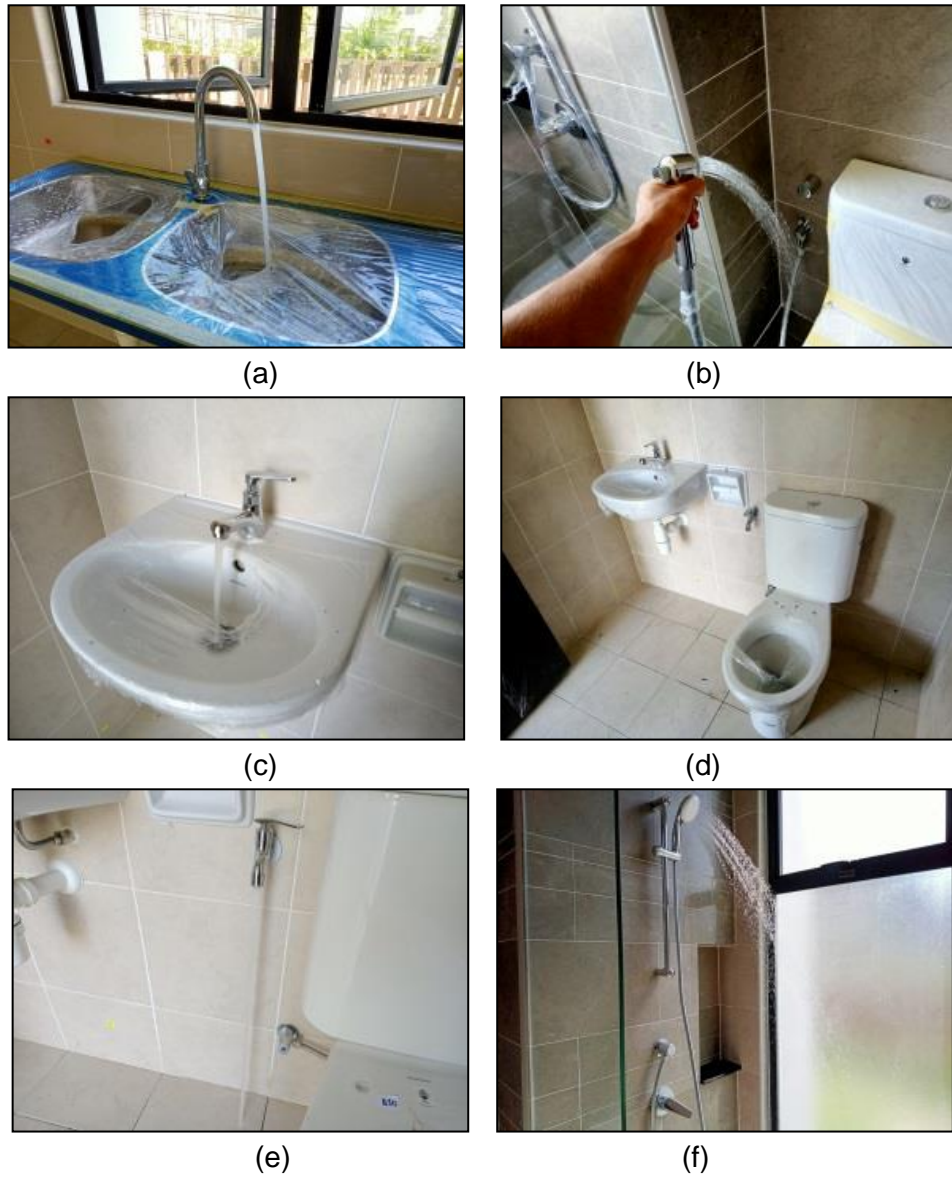
Figure 3.46 (a), (b) (c), (d), (e), (f): Sanitary and plumbing testing
