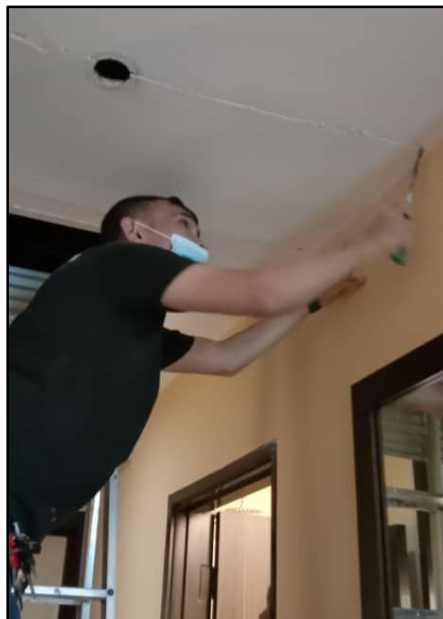
Figure 19: Cutting Ceiling
