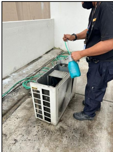
Figure 28: Cleaning Cooling Coil using Chemical Substance
