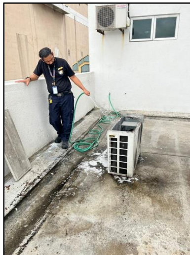
Figure 29: Cleaning Chemical Substance using Water
