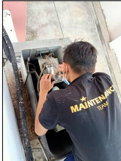
Figure 30: Capacitor Testing Process
