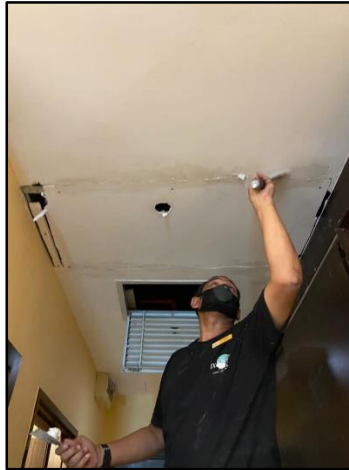
Figure 23: Plastering Work
