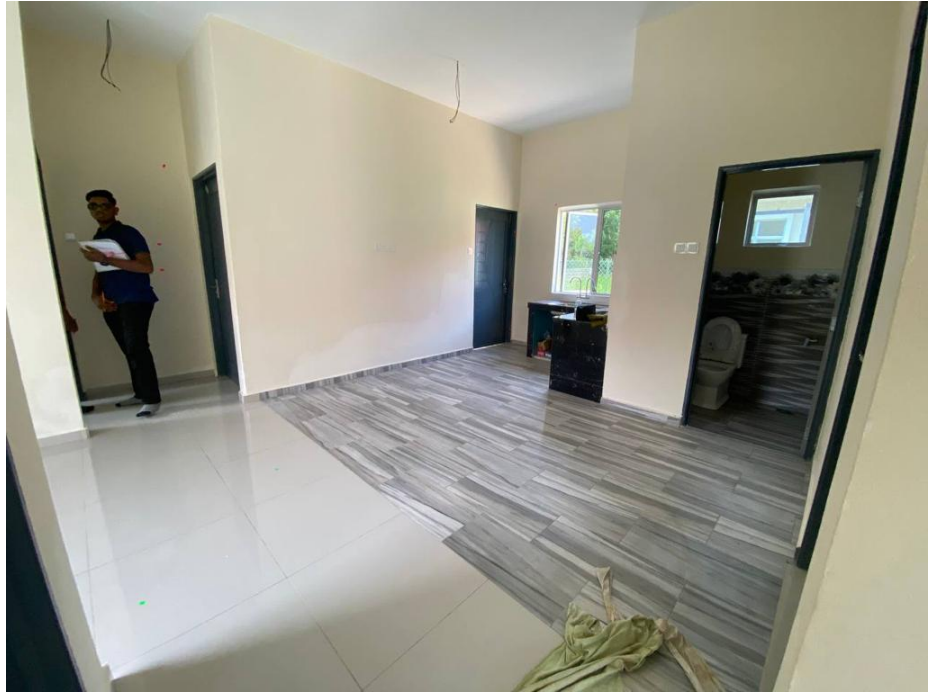
Figure 3.12 Inspection by main contractor
