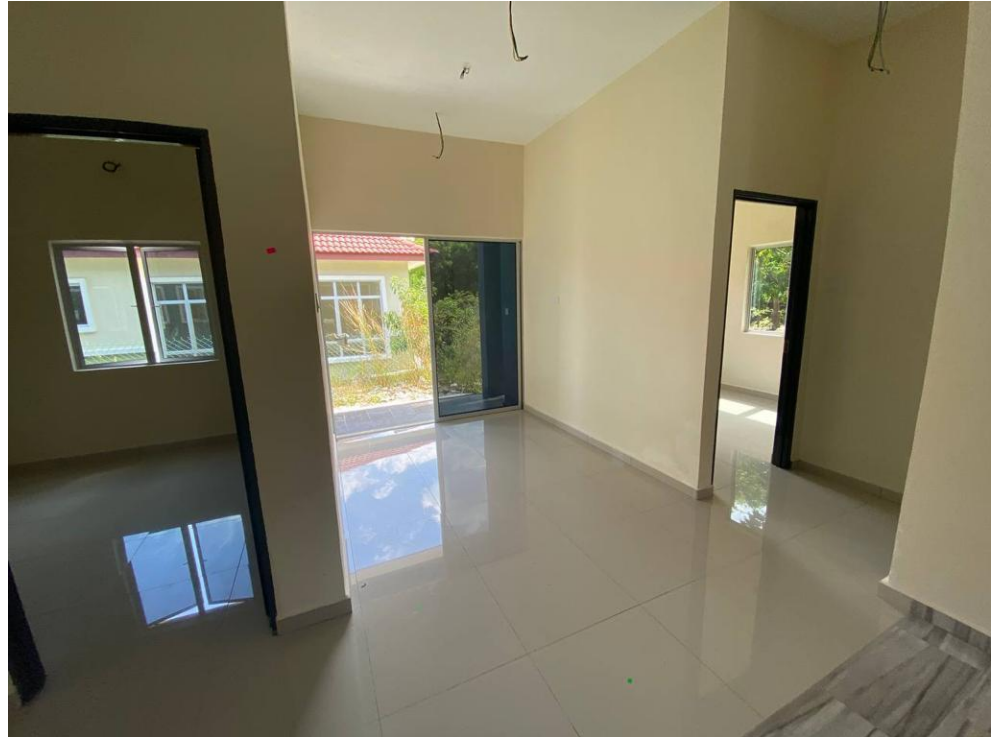
Figure 3.9 Inspection by client
