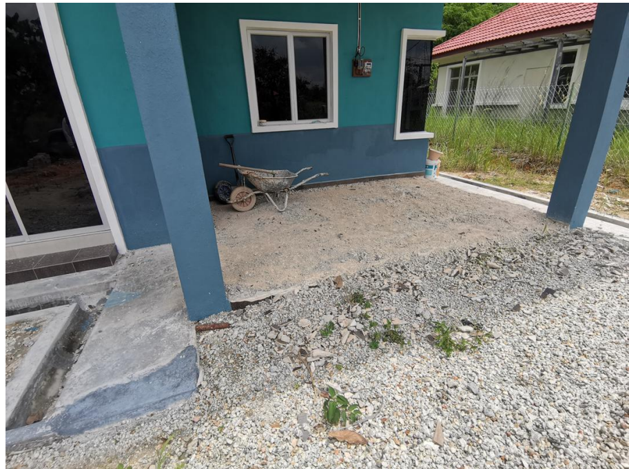
Figure 3.17 Repair in progress
