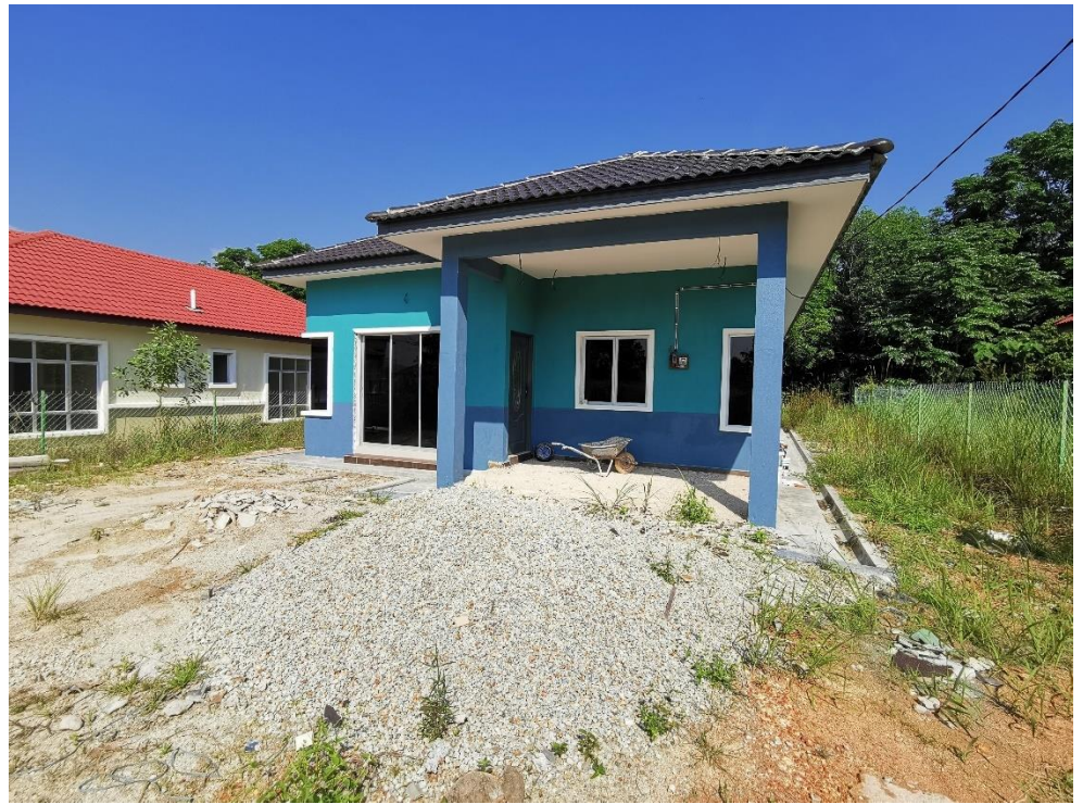
Figure 3.8 Inspection by client
