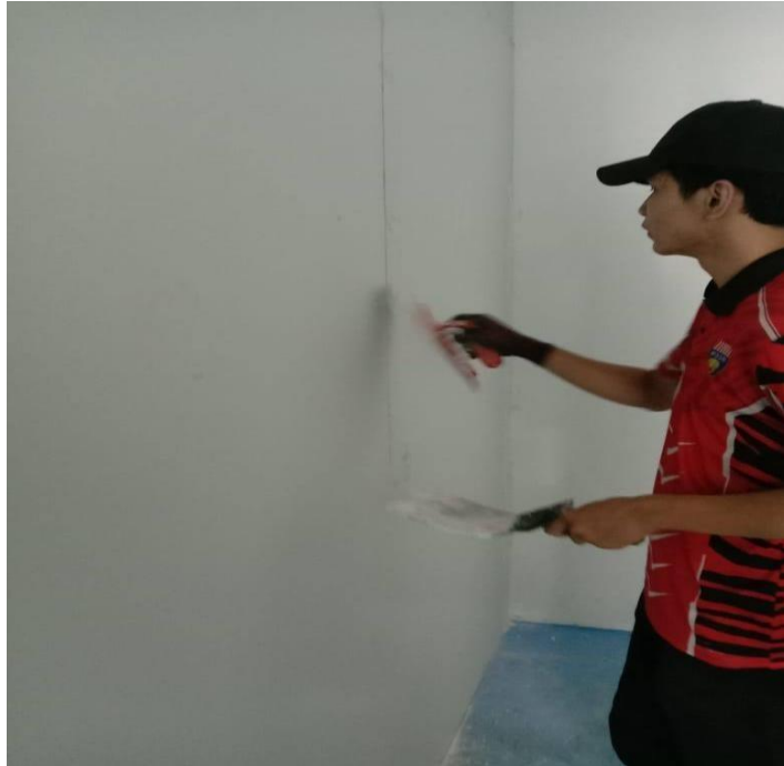
Photo 3.6: Plastering the wall surface
