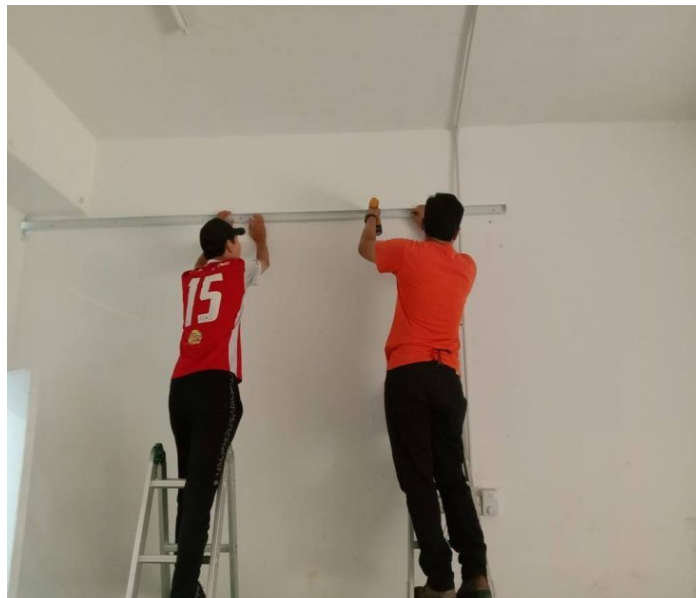
Photo 3.1: wiring works at subang
