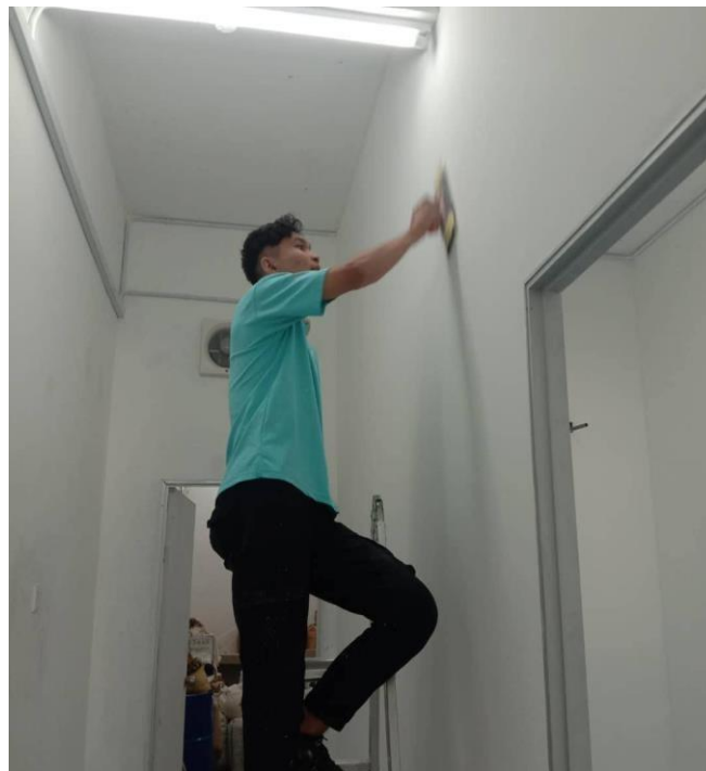
Photo 3.8: Ongoing partition wall installation
