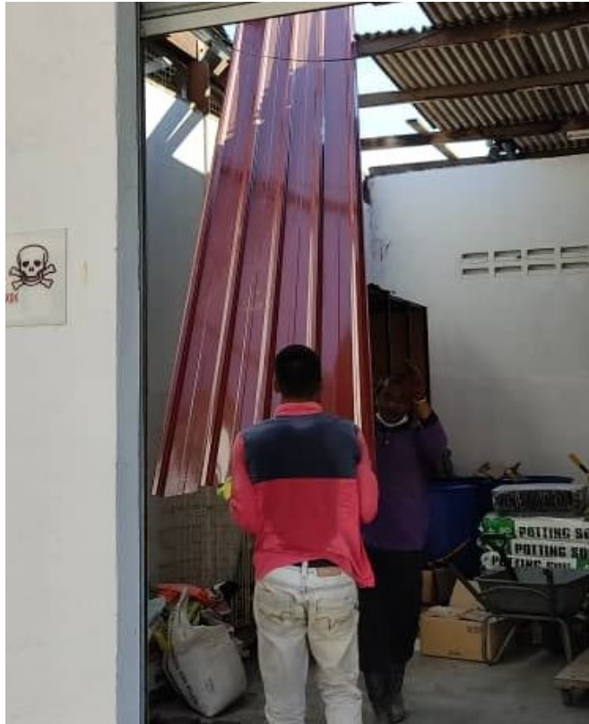
Figure 3.10: Roof removal process
