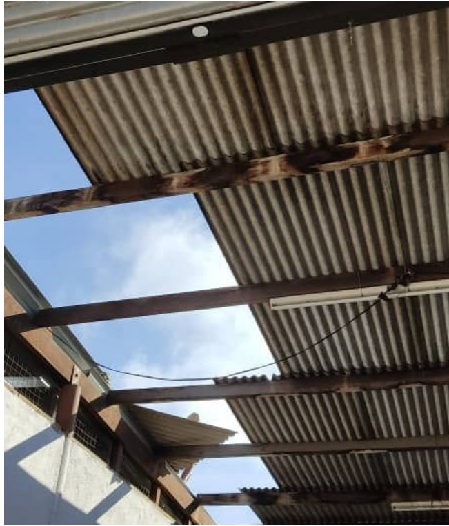
Figure 3.8: Condition of the roof during replacement work
