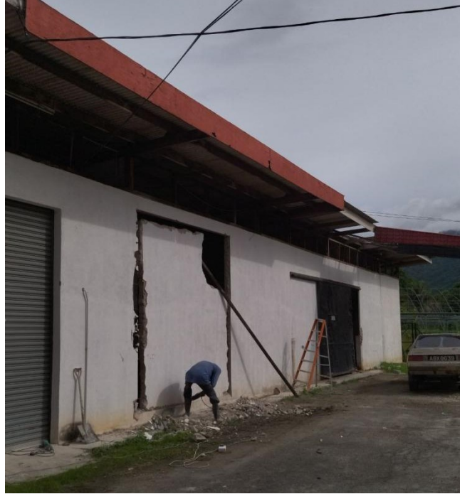
Figure 3.6: Demolition of wall
