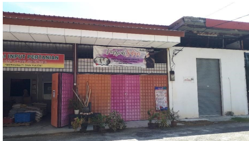
Figure 3.2: Adjacent of the building
