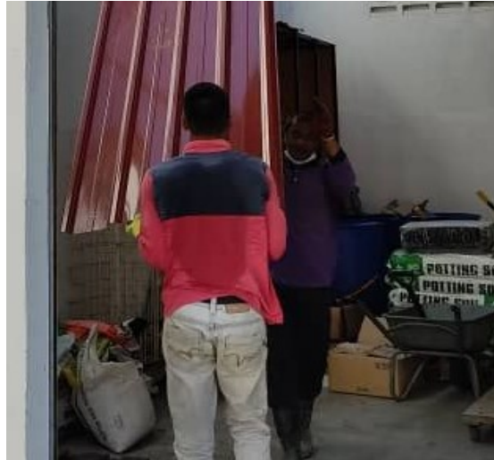
Figure 4.1: Process of moving the old roof
