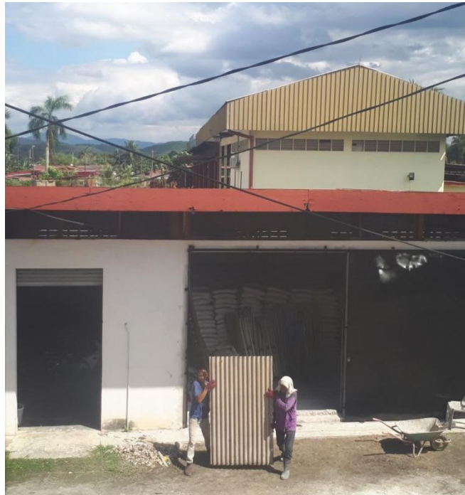
Figure 3.9: Roof removal process
