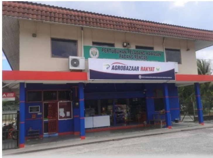
Figure 1.1: PPK Padang Rengas Building
