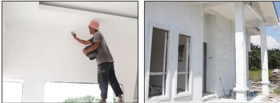
*Photo 3.14: Under-coat Work Process*
