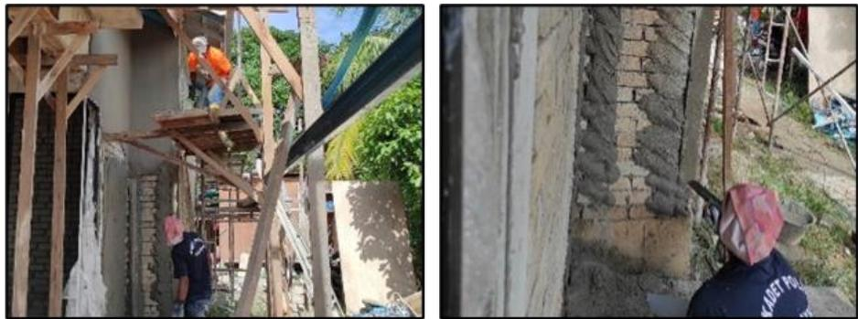
*Photo 3.8: Plaster Installation Process*
