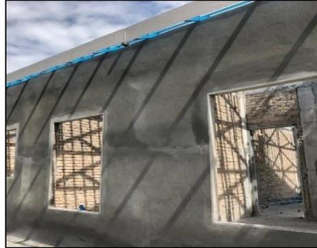
*Photo 3.7: Inspection of Plasterwork Process*
