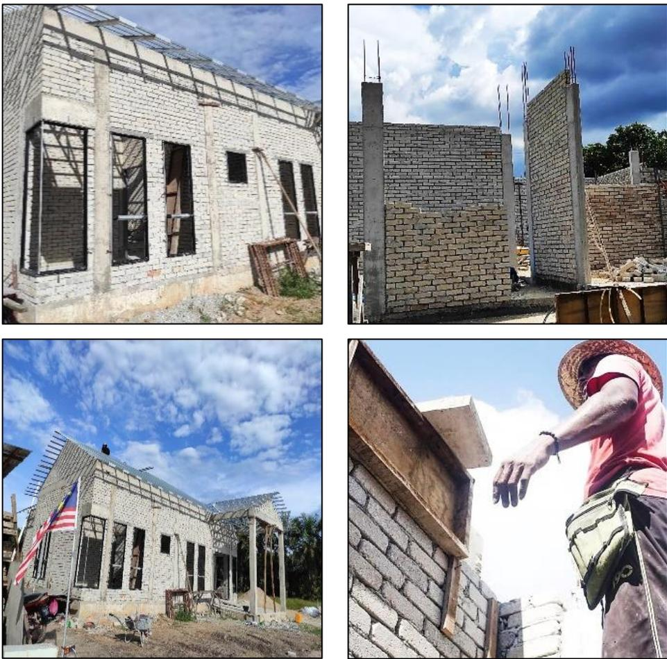
*Photo 3.6: Bricklaying Process*
