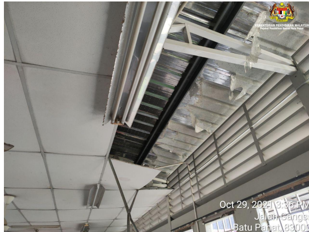
Figure 3.2.1 Damaged ceiling
