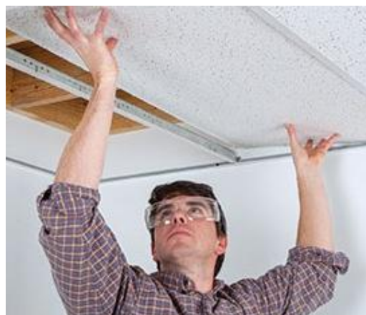
Figure 4.3.3 Placing the ceiling tiles
