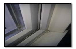
Figure 16: Window Cannot Close Properly
