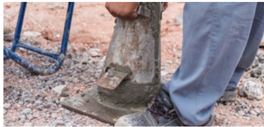
Figure 3.9: The placing of fresh concrete in the mold
