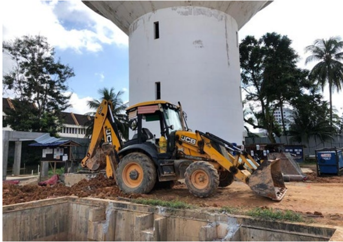
Figure 3.8: A bulldozer one of the machineries used
