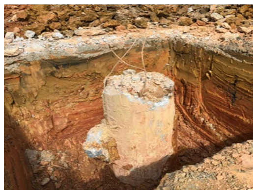
Figure 3.14: The excavation around pile
