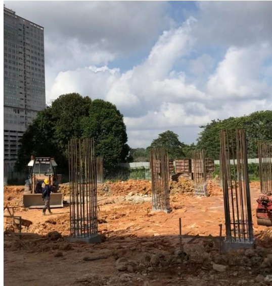
Figure 3.5: View of the project at 7% progress.
