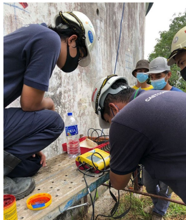
Figure 1.1: An observation of testing the thickness of pipe.
