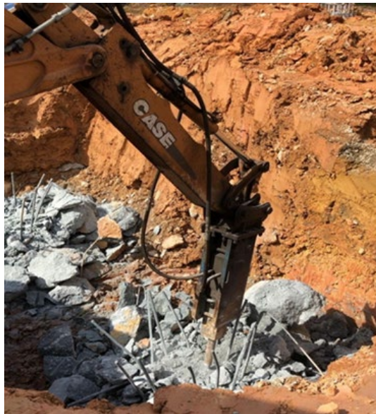
Figure 3.15: The cutting of the pile
