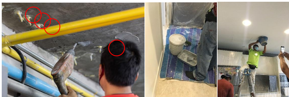
Figure 3.2.4m, n & o: Rectify leaking issue by PU injection
