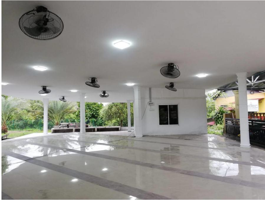
Figure 3.22 Installation of ceramic tiles is done
