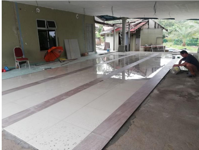
Figure 3.21 Installing the ceramic tiles
