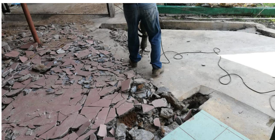
Figure 3.14 Workers are using jet hammers.
