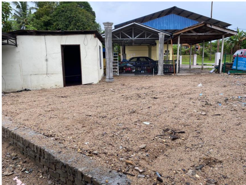
Figure 3.15 The condition of the finished floor sand is levelled
