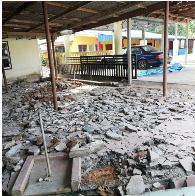
Figure 3.13 Ceramic tiles been demolished
