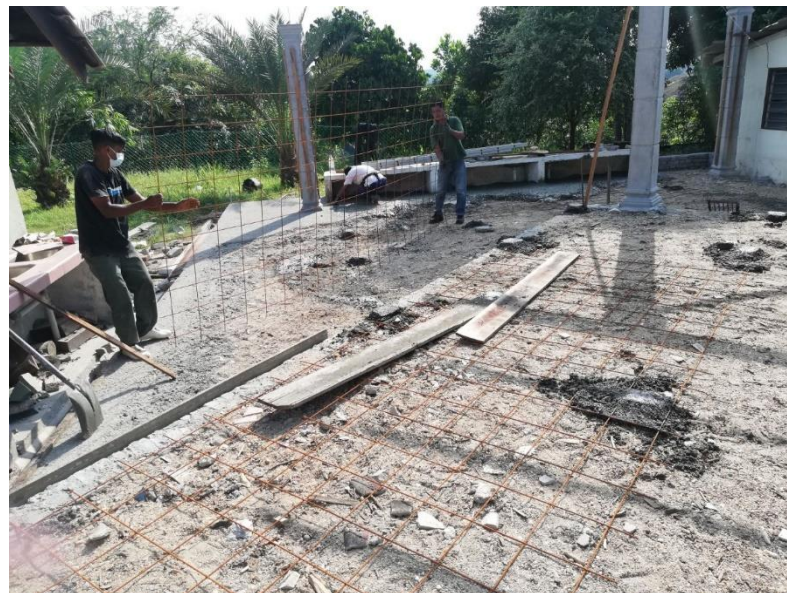
Figure 3.16 The worker are installing the BRC steel
