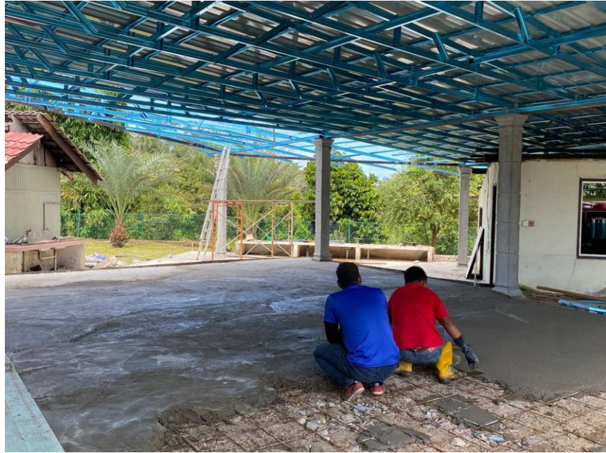
Figure 3.18 Workers are levelling the concrete floor
