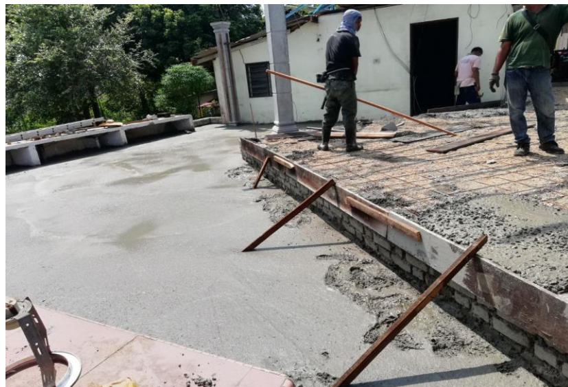
Figure 3.17 Bottom area were concrete
