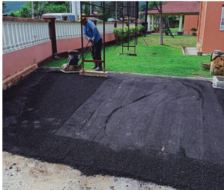
Figure 3.7: Spread the penetration grade bituminous base layer.
