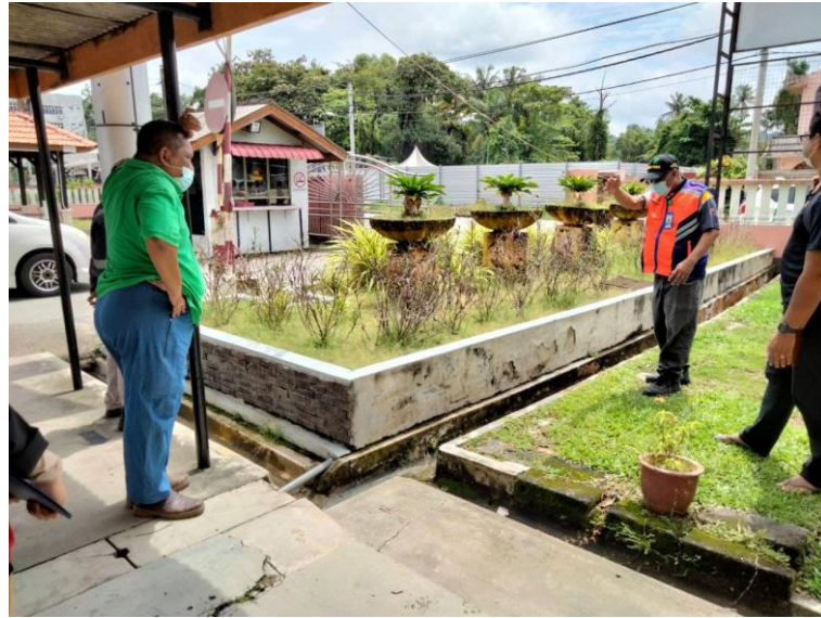
Figure 3.2: Site inspection of blockage pipe area.
