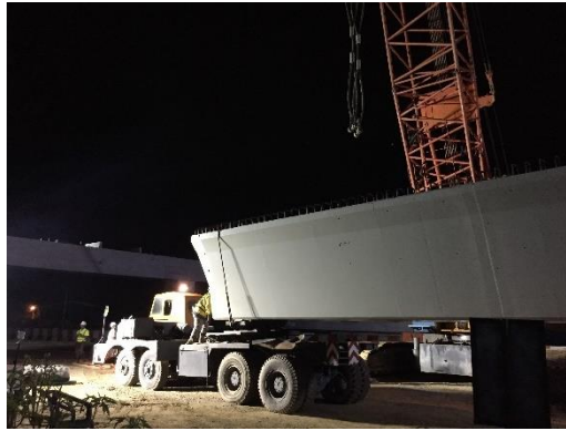
Figure 3.12: Prime movers' movement from the yard to the launching area.
