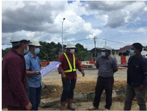
Figure 3.22: Inspection from the Jabatan Kerja Raya (JKR).
