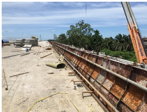
Figure 3.19: Concreting work for the precast parapet.
