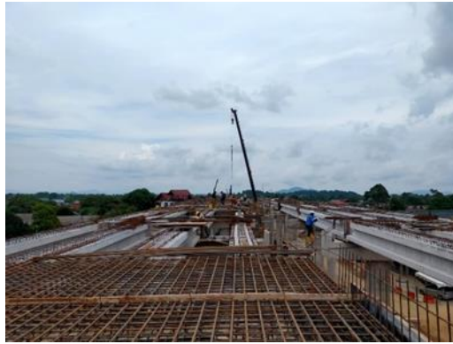
Figure 3.16: Installation of high tensile reinforcement bar.
