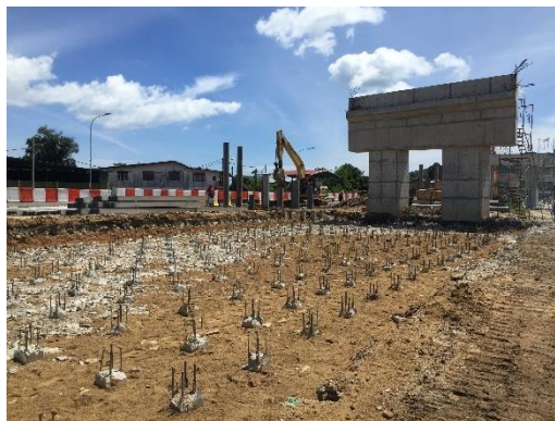
Figure 3.9: Pile embankment after the hacking process.
