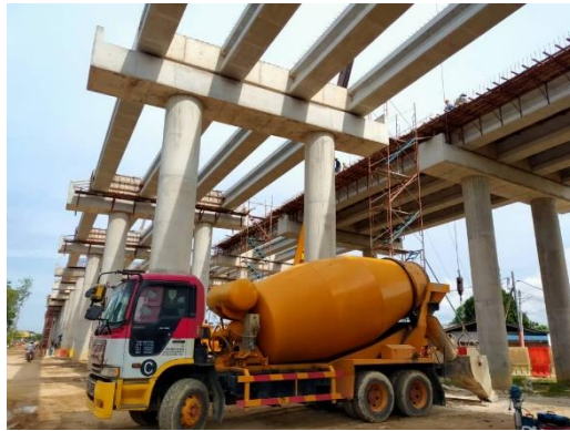
Figure 3.31: Concrete Mixture Transport Truck.
