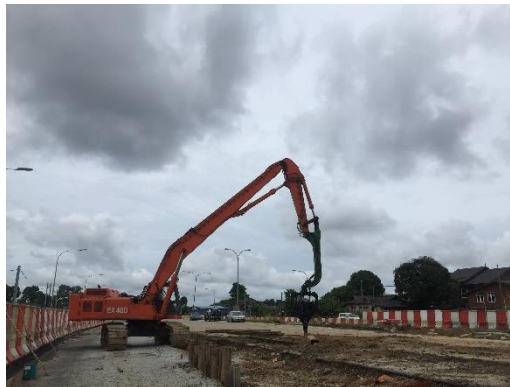
Figure 3.35: Sheet Pile Driving Machine.
