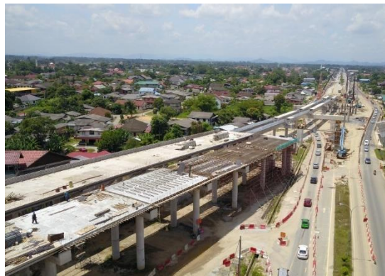
Figure 3.15: Drone view for the completed beam launching.
