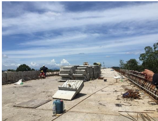
Figure 3.18: Installation of the precast parapet.
