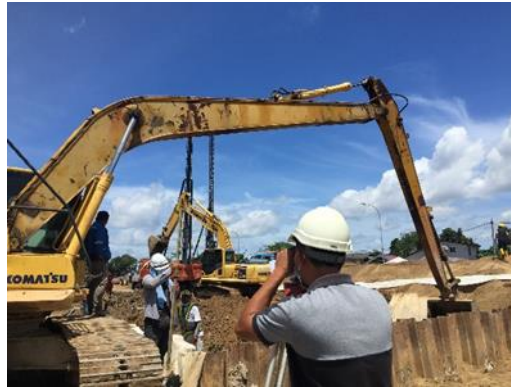
Figure 3.3: Site engineer is checking the excavation level.
