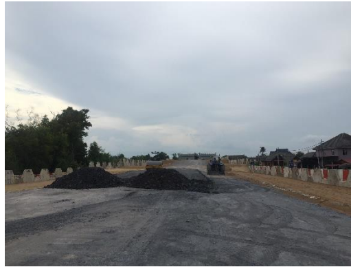
Figure 3.20: Layers of the soil for surfacing process.
