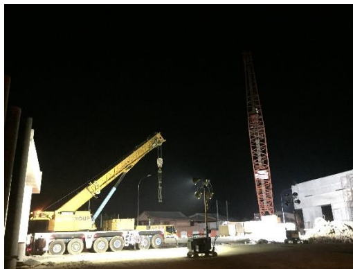
Figure 3.13: Beam launching process at the first span.
