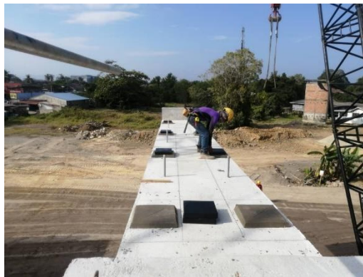
Figure 3.10: General worker is installing the bearing pad.
