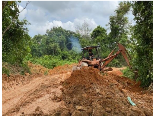
Figure 3.1: Site clearance process to demolish existing tree.
