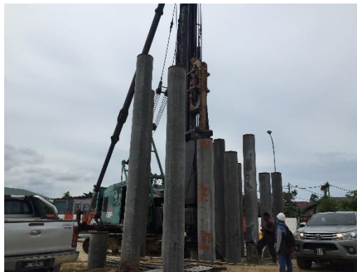
Figure 3.6: Piling injection using hydraulic hammer.
