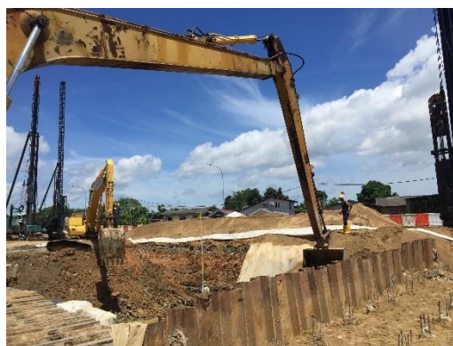
Figure 3.2: A 360-degree excavator is digging out the asphalt road surface.
