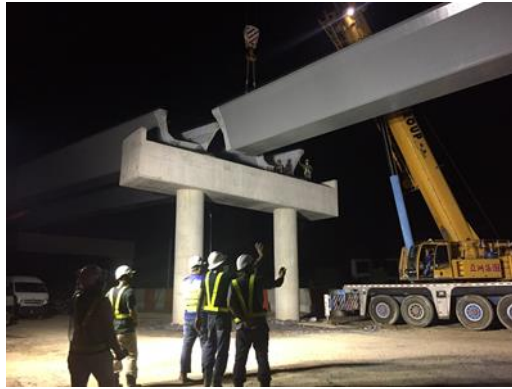
Figure 3.14: The general workers are adjusting the bearing pad by the help of site engineers.
