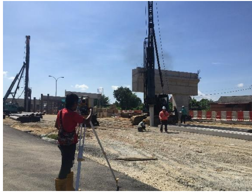
Figure 3.5: The surveyor is aiming crosshairs for piling level.
