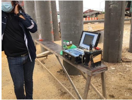
Figure 3.7: Observing the data analysis for the Pile Driving Analysis Test.
