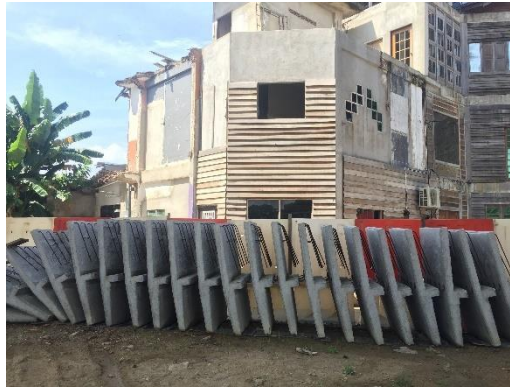
Figure 3.17: Precast parapet that was placed under the bridge.
