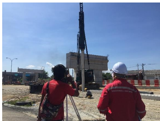
Figure 3.4: Surveyor is taking the level for piling.
