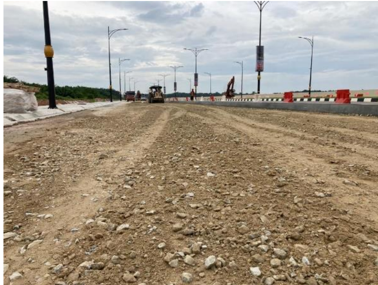
Figure 3.6: Crusher run at Zone 2.1
