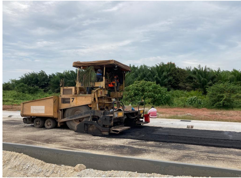
Figure 3.7: Premix works at Zone 2.1
