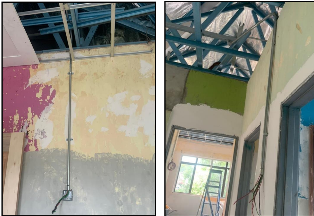
Figure 5: The electrical work at the quarters.
