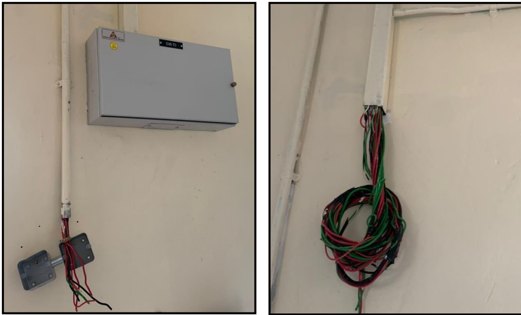
Figure 4: The work that need to do maintenance at PHN
