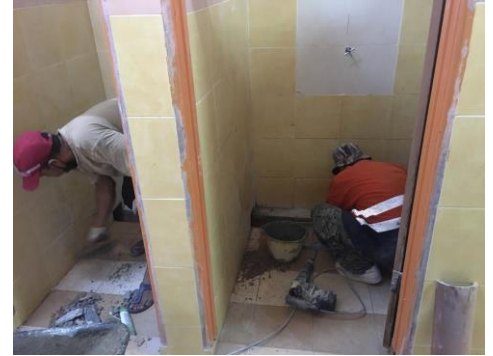
Figure 20: Install the half round clay drains
