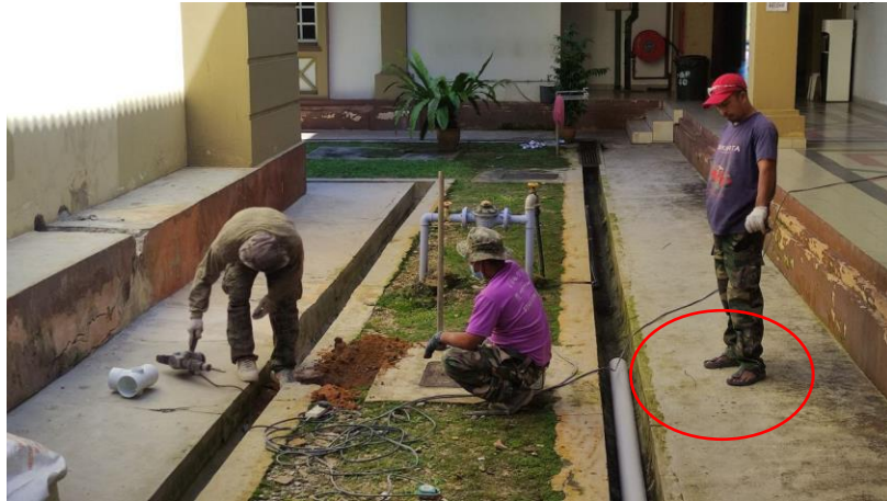
Figure 24: Drilling work at manhole
