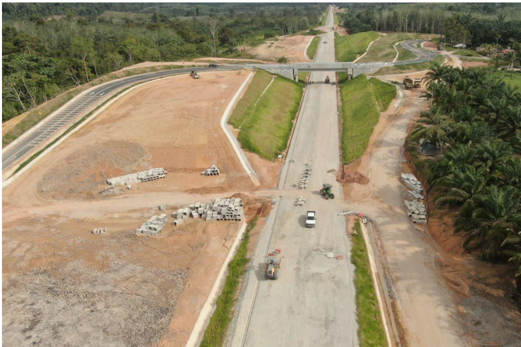
Figure 1.1: Overview for earthworks of railway track
