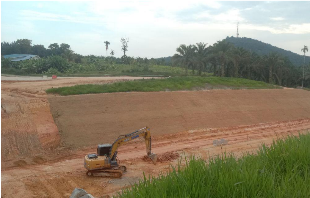
Figure 3.2: Site clearing at Kampung Lenek, Bekok
