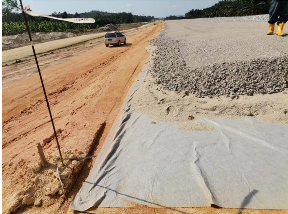
Figure 3.4: Laying geotextile and sand blanket
