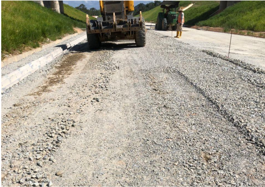
Figure 3.5: Laying sub ballast and ballast
