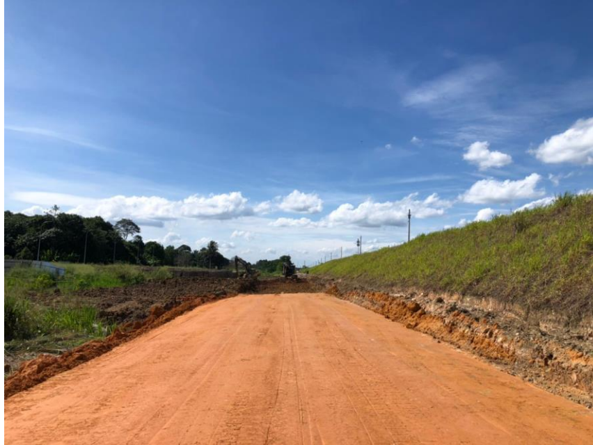
Figure 3.3: Earthworks (subgrade and embankment fill)
