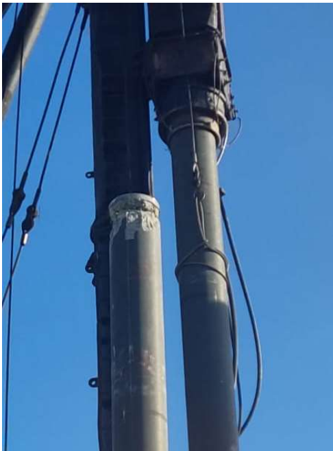
Figure 3.3.1 Head Crack
