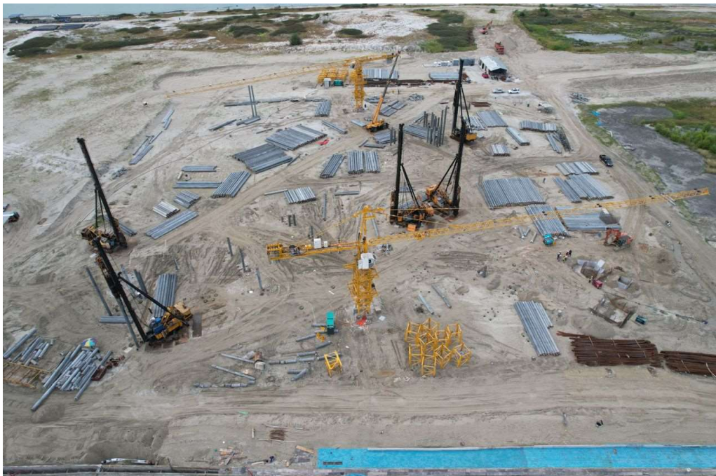
Figure 3.1.7 Piling Works
