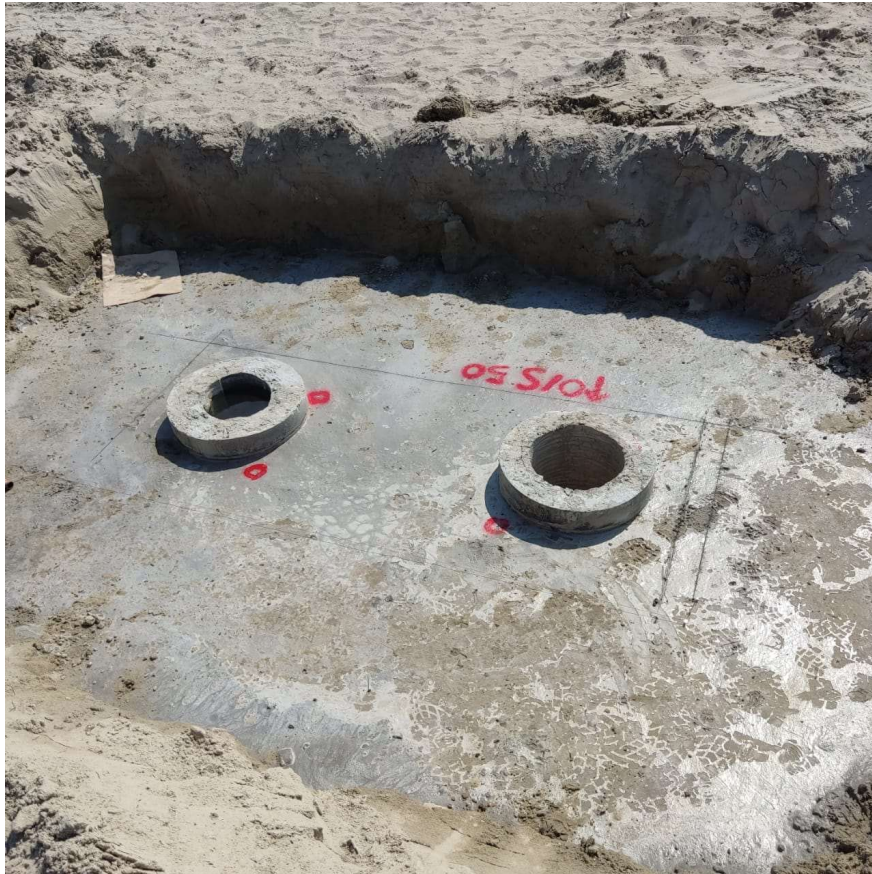
Figure 3.4.3 Pile Cap Concrete
