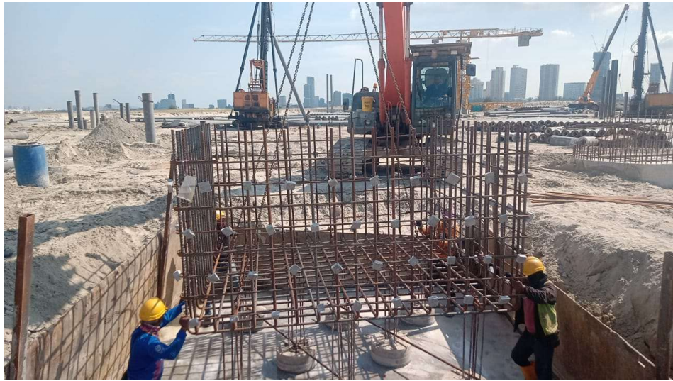
Figure 3.4.2 Install Pile Cap Rebar
