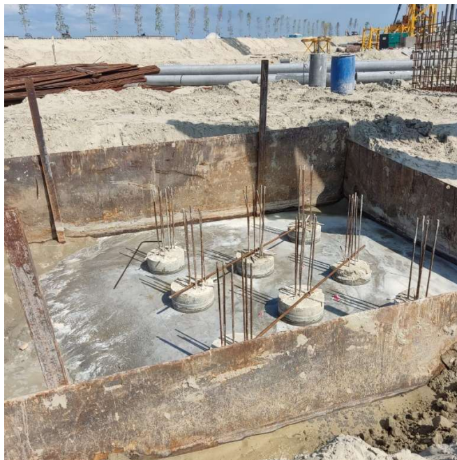
Figure 3.4.1 Pile Cap Detail
