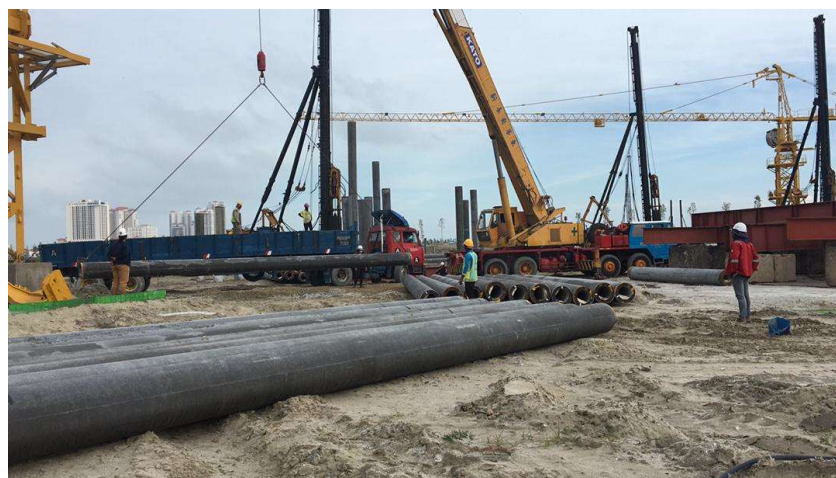
Figure 3.2.2.2 Unload Pile
