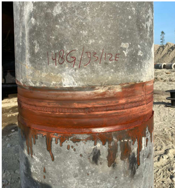
Figure 3.2.1.1 Pile Welding Joint
