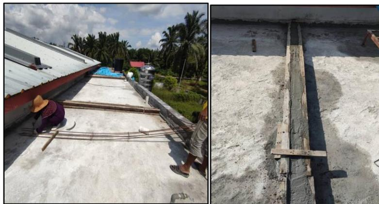
Photo 3:31 Process of create divider beam
