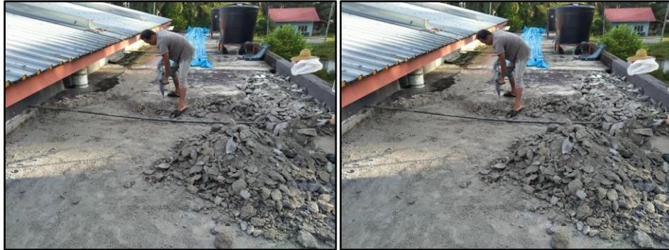
Photo 3:27 Process of hacking work
