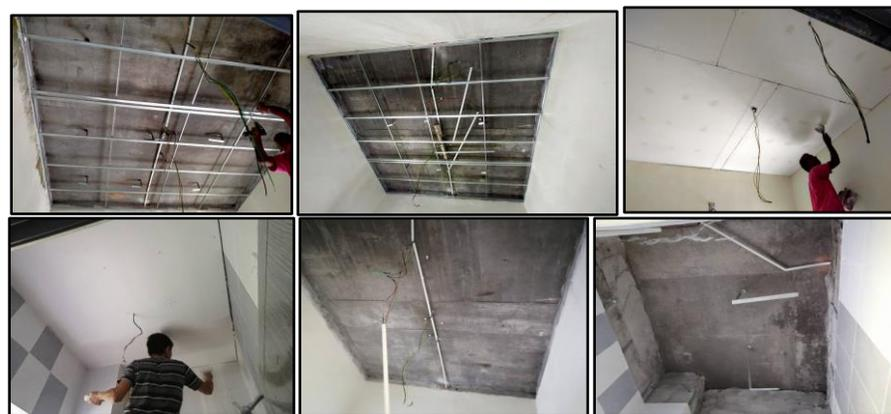
Photo 3:35 Process of ceiling installation
