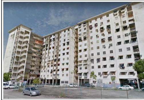
Figure 1.3: The Front View of Block A
