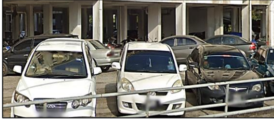
Figure 1.21: Car Park Block A
