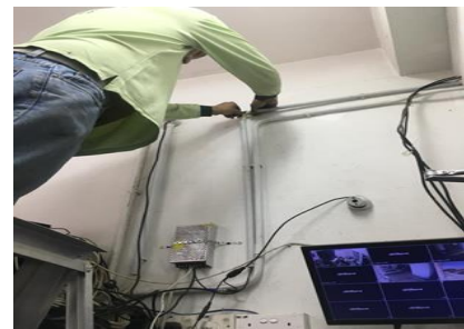
Figure 3.37: Setting up the wiring of CCTV at office.
