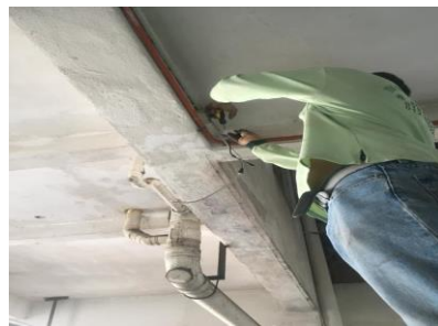
Figure 3.36: Install the bluetooth at Block A and B
