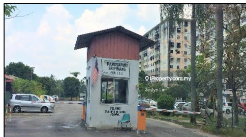
Figure 3.34: Guard House of Block B and C
