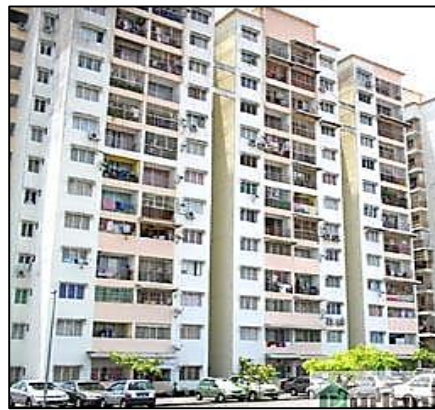
Figure 1.5: Show the Front View of Block B
