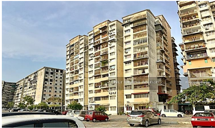
Figure 1.1: Taman Sri Pinang Apartment, Pulau Pinang
