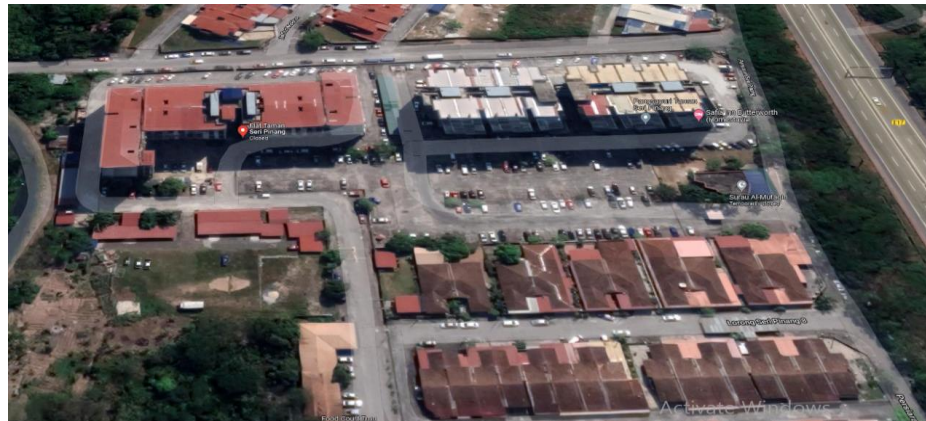
Figure 1.12: The View Adjacent Building Surrounding Area Apartment TSP
