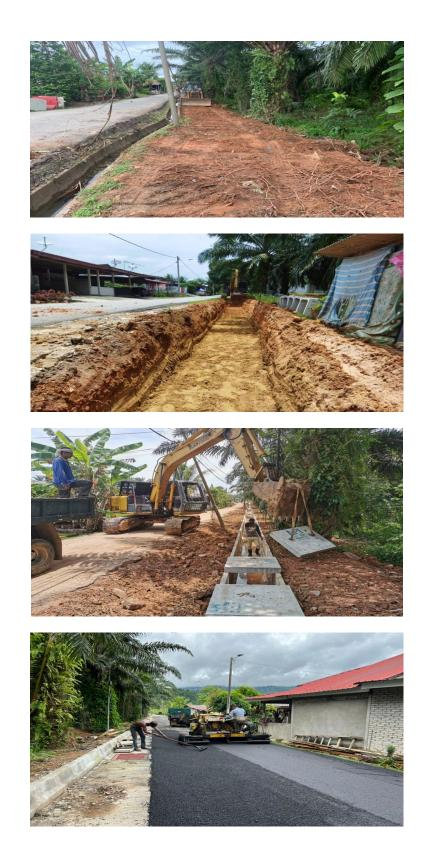
Figure 8 : During road widening works in RPT Gua Badak, Lenggong
