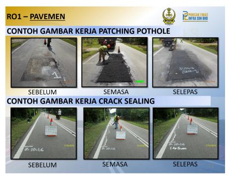
Figure 14: On-site work for patching pothole and crack sealing
