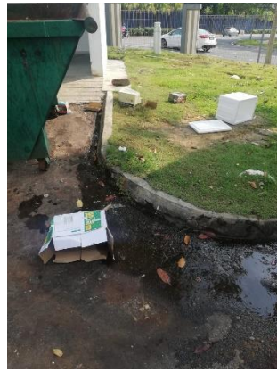
Figure 3.42: Stagnant water at leaking pipe area
