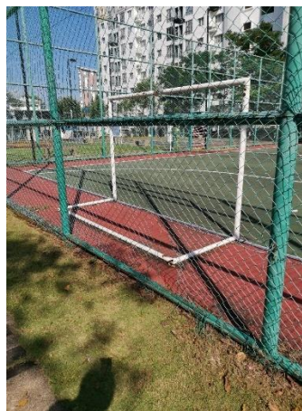
Figure 3.59: Condition one of the wire fences after the work
