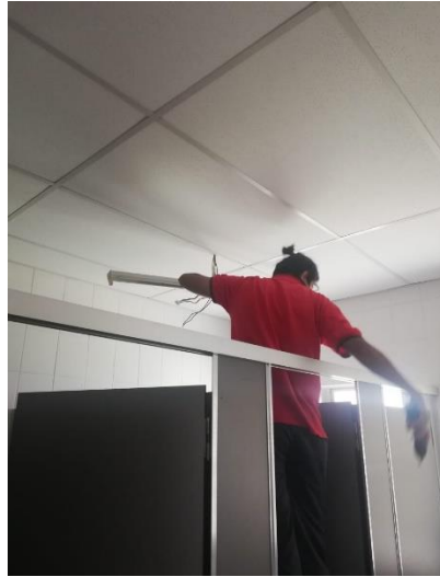
Figure 3.54: Rewiring work to use LED lamp
