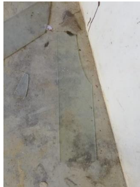
Figure 3.39: Broken glass window
