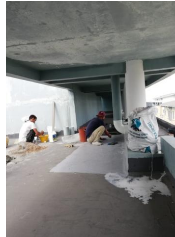
Figure 3.37: Laying new waterproofing and adjust the direction of rainwater down pipe
