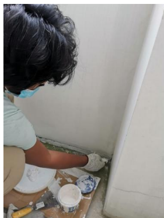
Figure 3.48: The used of filler to close the minor crack
