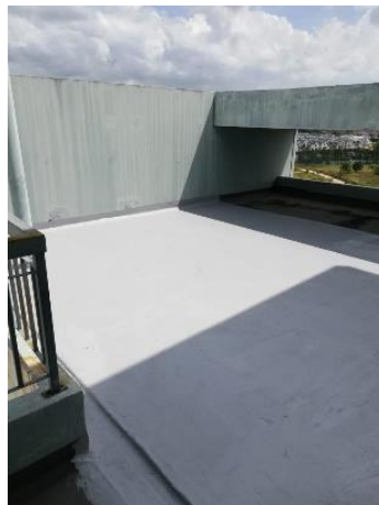
Figure 3.35: Condition of the new waterproofing after fully dry
