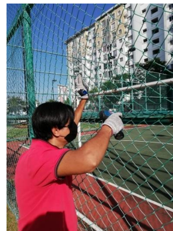
Figure 3.58: Install new screw by using the impact driver cordless
