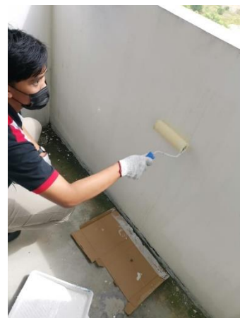
Figure 3.49: First layer of re-painting work
