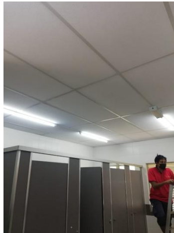
Figure 3.56: Result after the process of replacement is done
