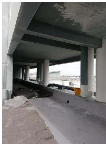
Figure 3.38: The condition after the repairing work done
