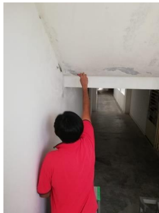
Figure 3.46: Scrap all loose paint at staircase
