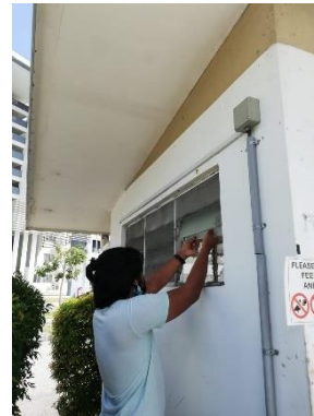
Figure 3.40: Replacement new glass window by the technician
