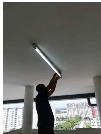
Figure 3.52: Adjust loose casing of LED lamp
