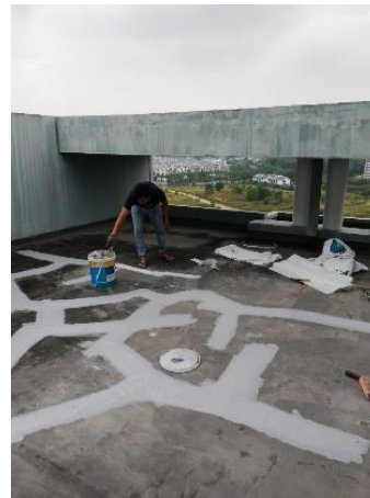
Figure 3.34: Laying new waterproofing (Quicseal 103)
