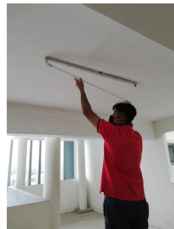
Figure 3.51: Replacement of LED lamp
