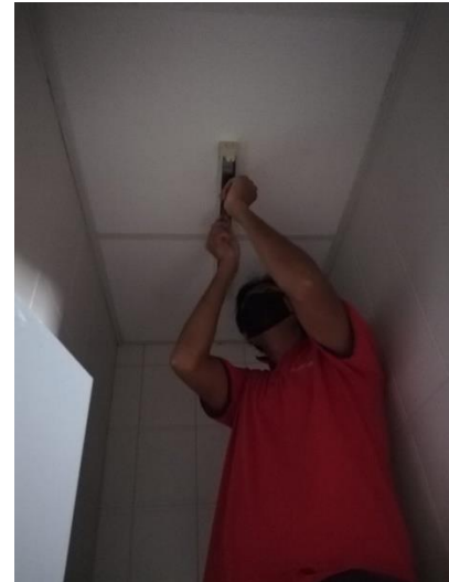
Figure 3.55: Different size of lamp use at the shower area
