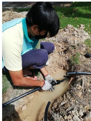
Figure 3.44: Install pipe connector to a new PVC pipe
