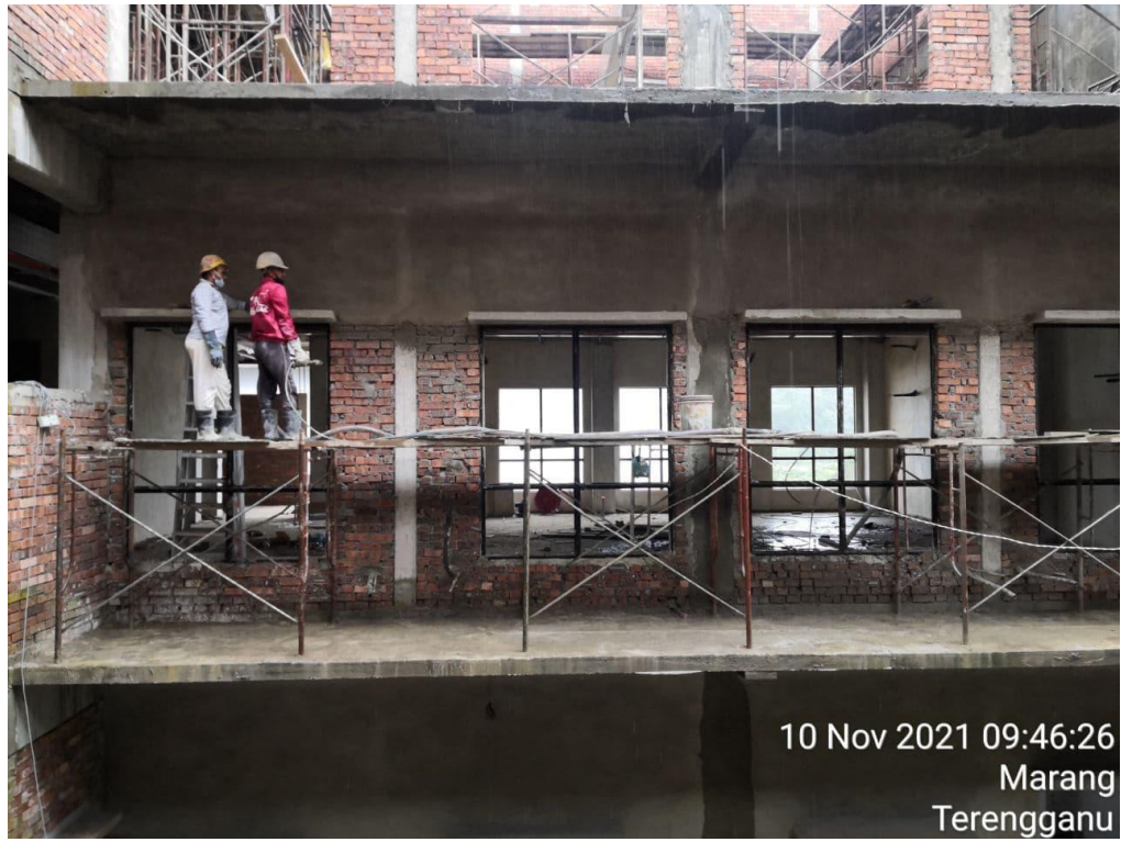
Photo 21: Mortar spraying
