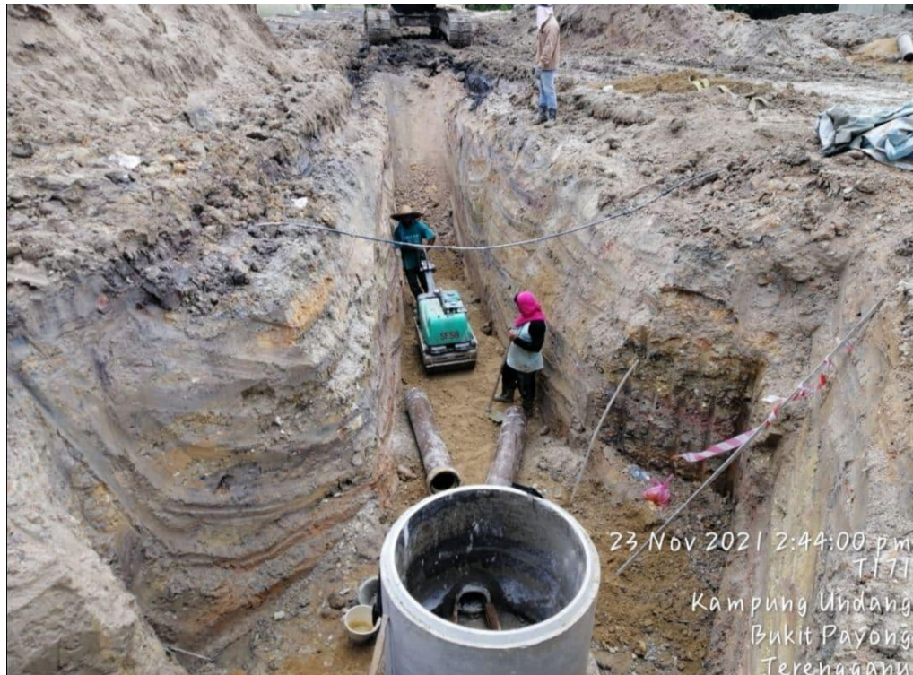
Photo 23: Compacting soil
