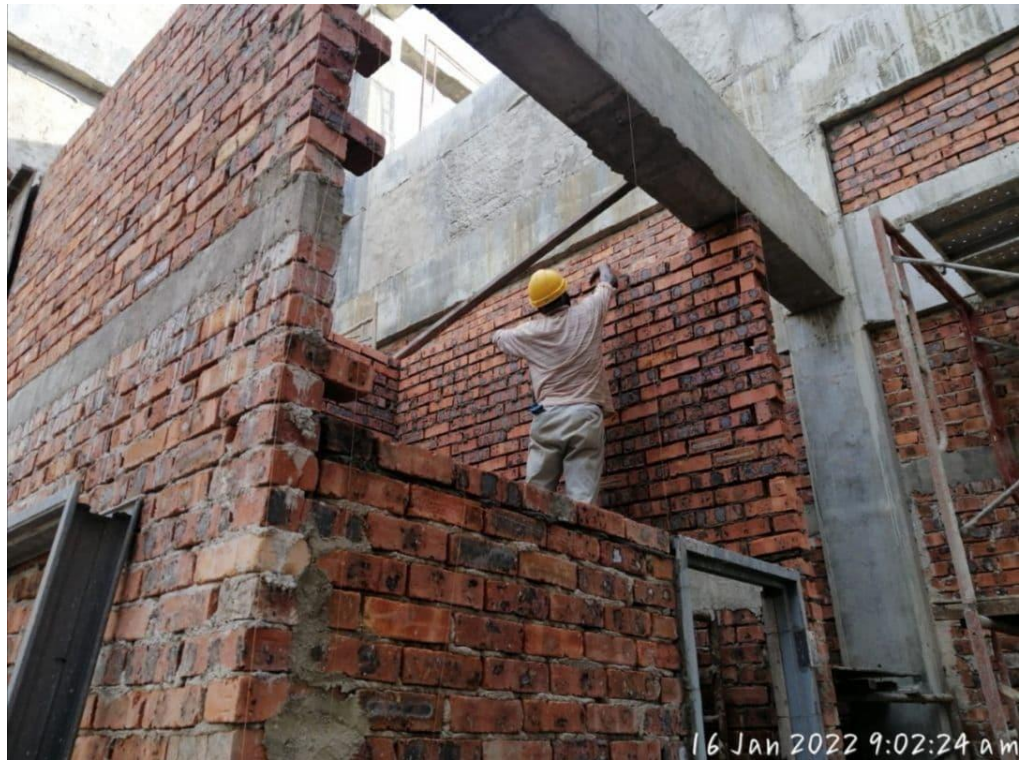
Photo 24: Brick walls installation
