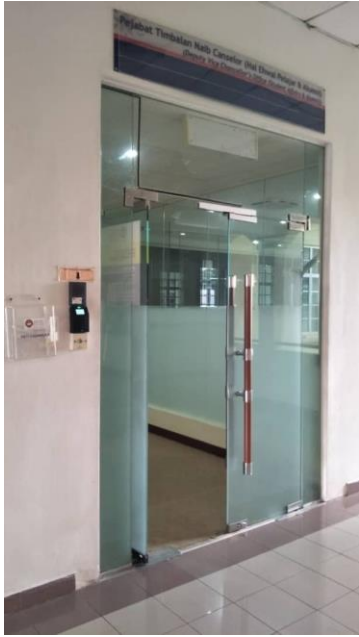
Figure 9 Existed Main Entrance Door
