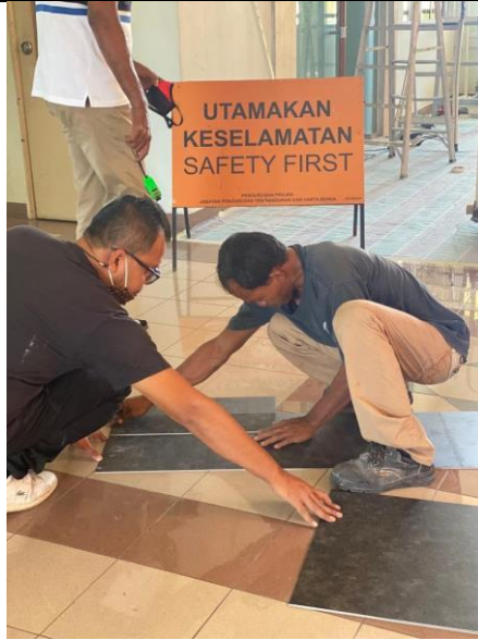
Figure 17 vinyl measure and cutting work
