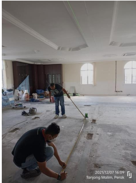
Figure 13 Setting off floor Partition wall Installation
