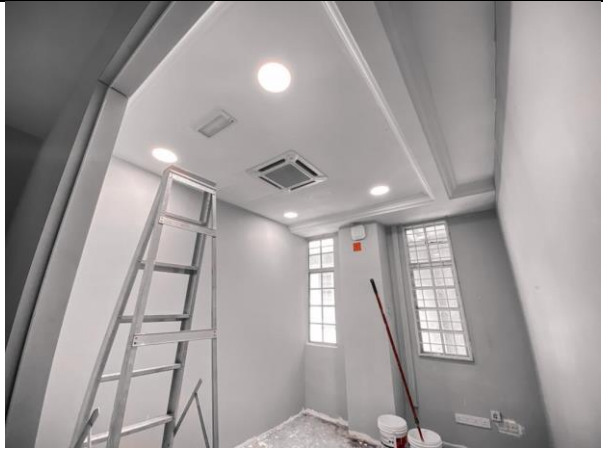
Figure 24 Complete ceiling and lamp installation
