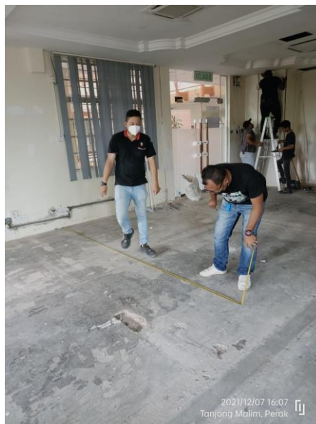
Figure 14 Setting off floor Partition wall Installation
