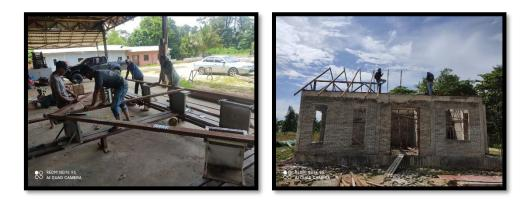
Figure 2 : Installation of wooden IBS at the factory and construction site
