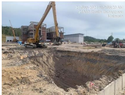
Figure 14: Excavation Work on STP
