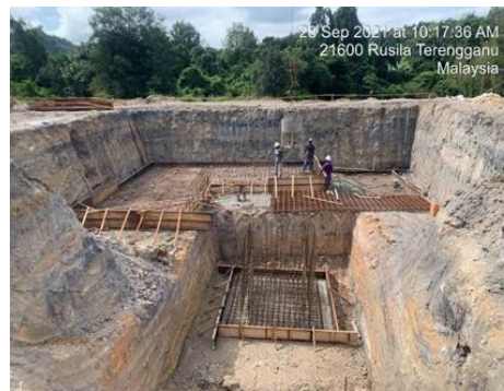
Figure 14: Excavation Work on STP
