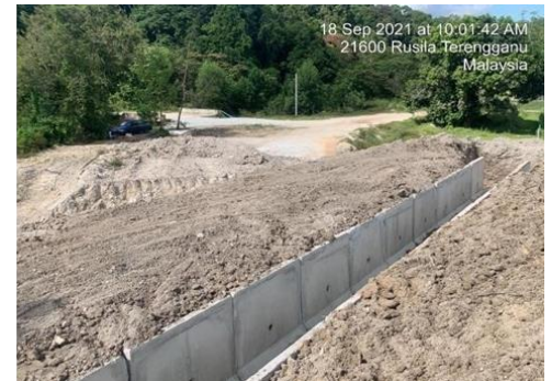
Figure 9: Pre-Cast U-Shape Drain
