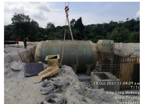
Figure 14: Excavation Work on STP
