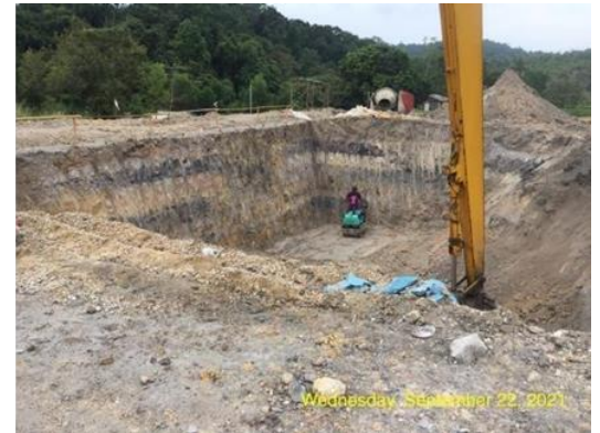
Figure 14: Excavation Work on STP
