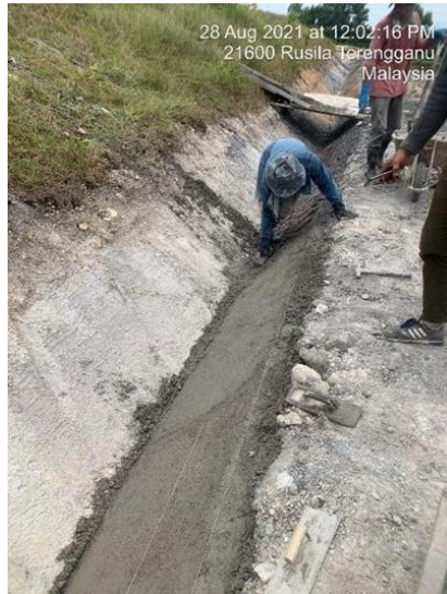
Figure 12: In-Situ V-Shape Drain
