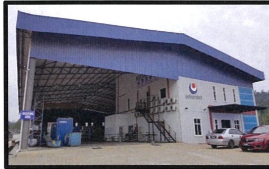
Figure 1: Solar Alert Sdn Bhd, Teluk Kalong Kemaman
