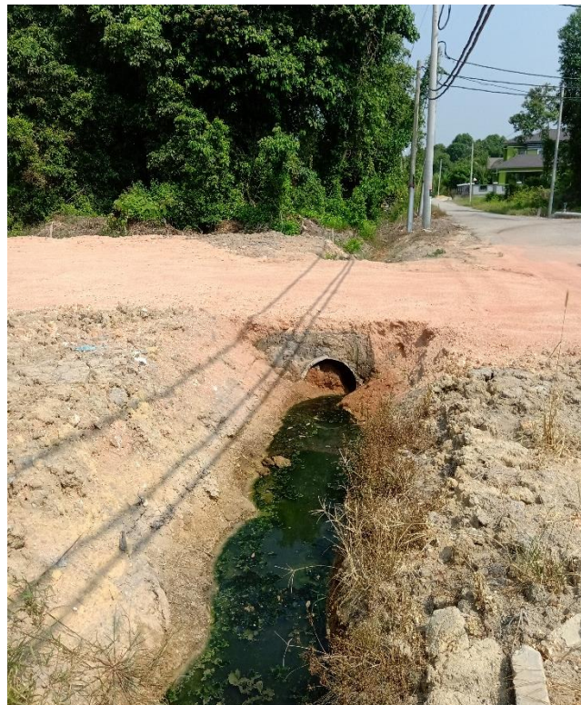
Figure 15: Roadside Drainage
