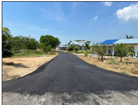
Figure 3.10: Result of the pavement at Kampung Raja Bashah
