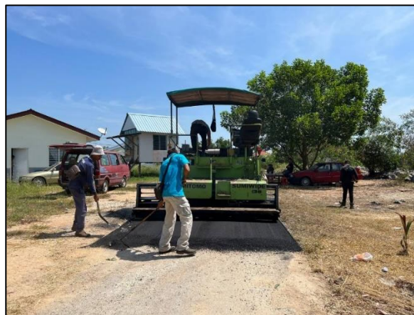
Figure 3.8: Lay wearing course using paver machine
