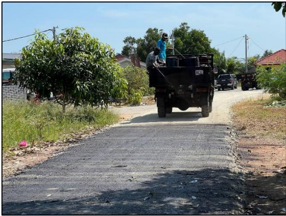
Figure 3.6: Tack coat during spraying process
