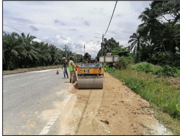
Figure 2.10: Tandem roller compaction
