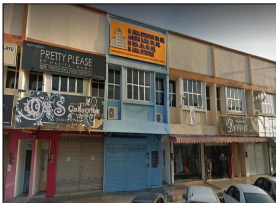
Figure 1.1: SK Juara Enterprise Sdn Bhd Building
