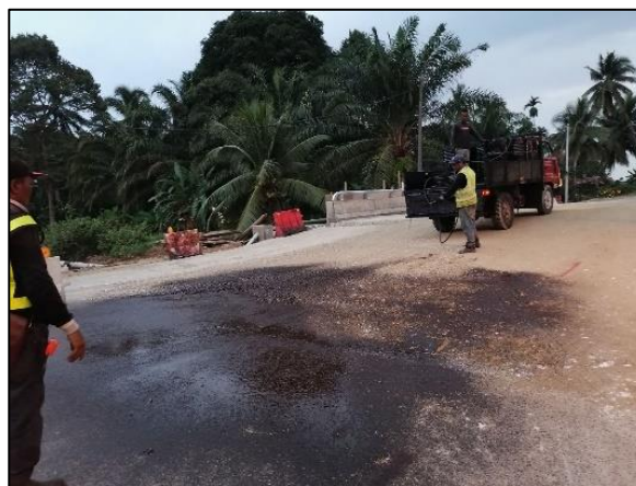
Figure 2.7: Application of prime coat
