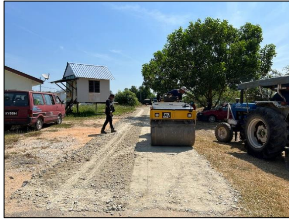
Figure 3.5: Tandem roller compact the crusher run
