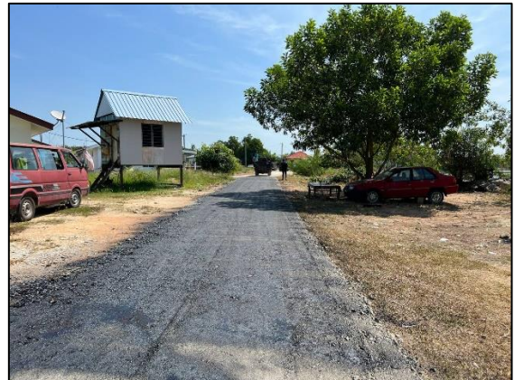
Figure 3.7: Tack coat after spraying process
