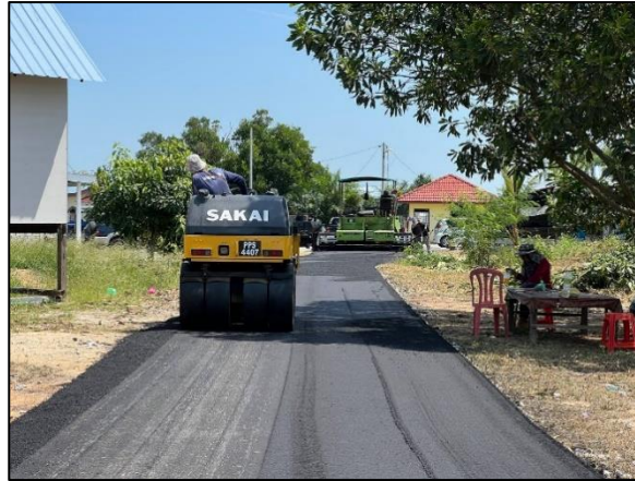
Figure 3.9: compaction premix using tandem roller 6tonnes
