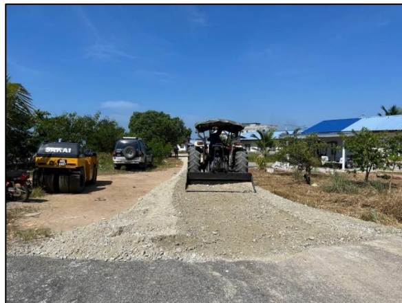
Figure 3.4: back pusher grading the crusher run
