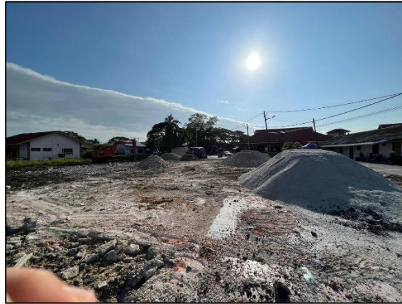
Figure 3.3: The stockpile of crusher run
