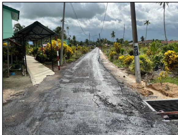
Figure 2.8: Application of tack coat
